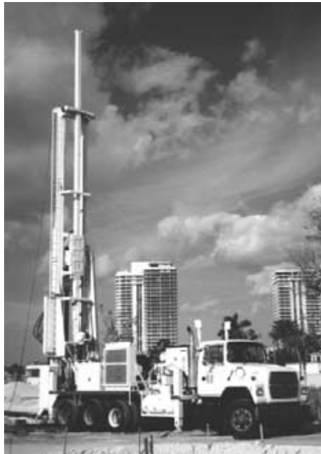
Figure 11-1: Dual rotary drilling rig used for shallow drilling (courtesy of Foremost Industries Incorporated).
