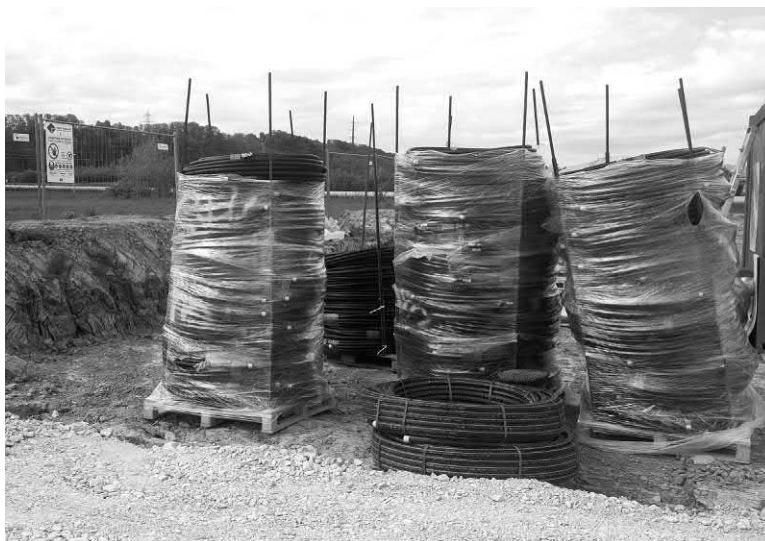
Figure 16.7 Stock of pipes in a dedicated portion of a construction site.
