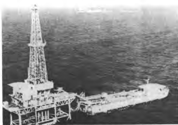
Fig. 1.12 – A tendered platform rig. 12
