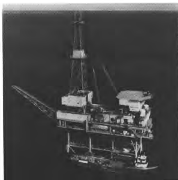
Fig. 1.11 – A self-contained platform rig on location in the Eugene Island area, offshore Louisiana.
