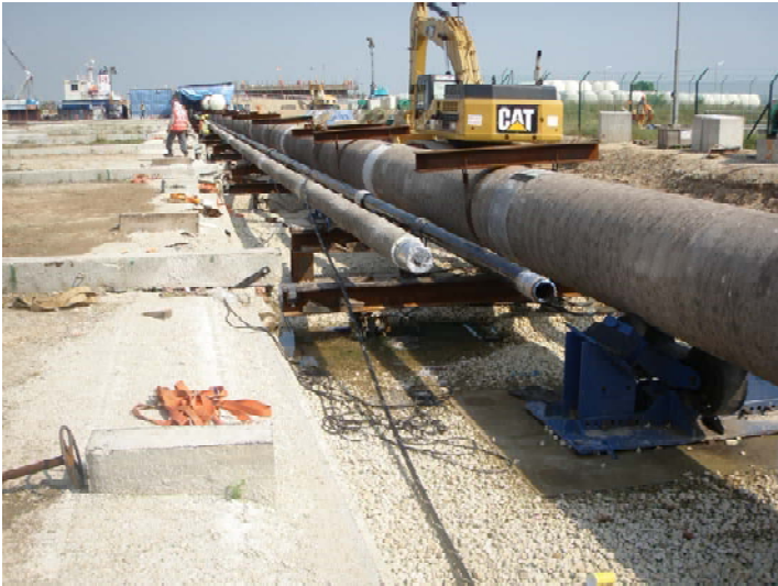
Figure 7.8 Bottom pull construction
