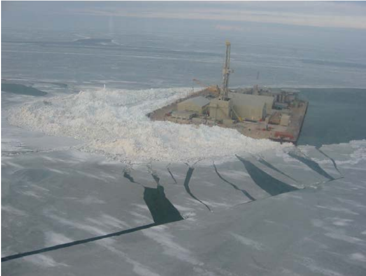
Figure 5.19: Ice rubble build-up around a shallow water platform (from [40]: photo by Derek Mayne)
