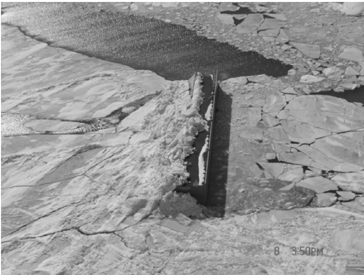
Figure 4.11 Sloping ice barrier in the Caspian Sea [44]
