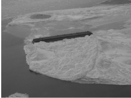
Figure 5.20 Rubble in front of a wide barrier (from [42]: photo by Rune Nilsen)
