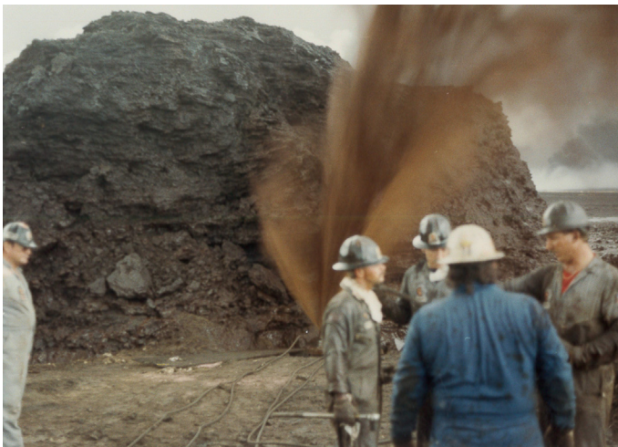
Fig. 11.8 Mound of coke had to be removed to get to the well.
