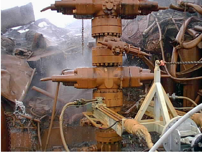
Fig. 6.29 Jet cutting (Courtesy of BJ Services.)
