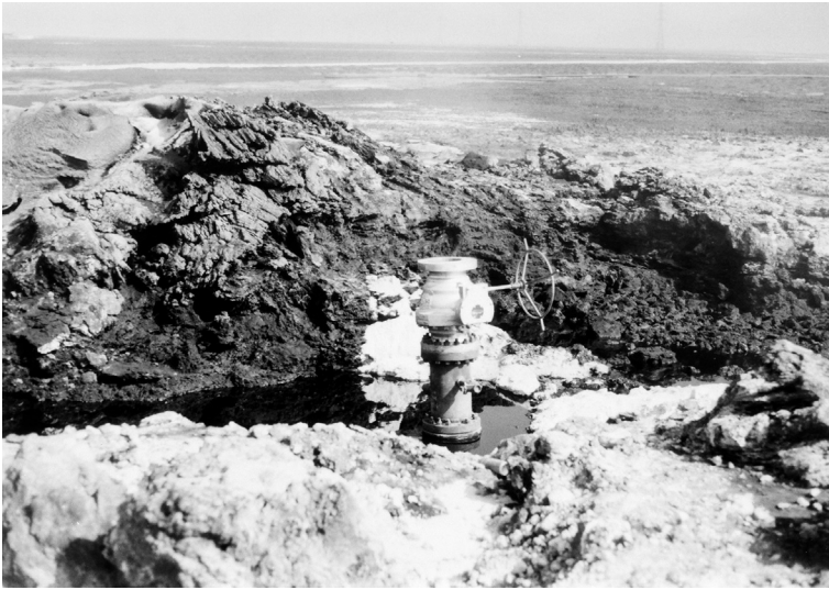
Fig. 11.13 Capping spool kill method.
