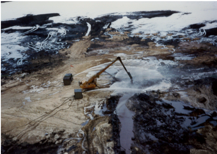
Fig. 11.11 Removing the coke pile and exposing the wellhead.
