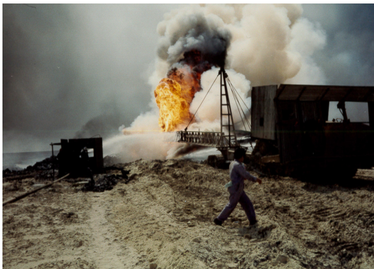
Fig. 11.18 Explosive charge being positioned for detonation in order to extinguish the fire.
