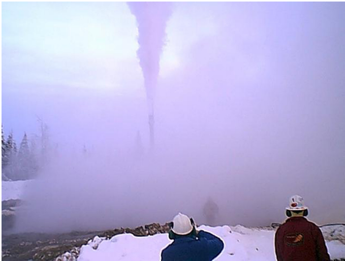
Fig. 6.28 Vision impaired while installing capping stack.
