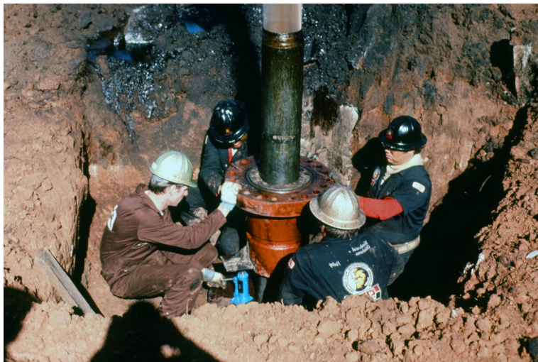
Fig. 6.26 Casing head slipped over casing and set with hydraulic jacks.
