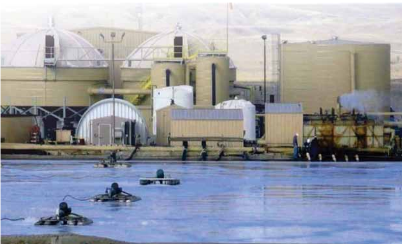
Fig. 6.10—Frac water lagoon and treatment plant (Boschee 2012).
