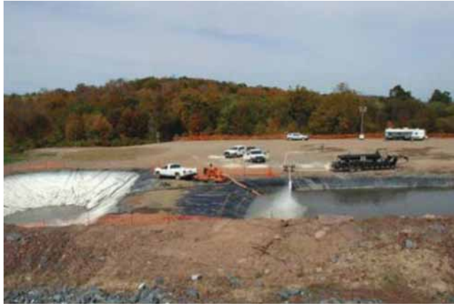
Fig. 6.7—Frac pit for flowback fluid collection (Tinto And Solomon 2010).
