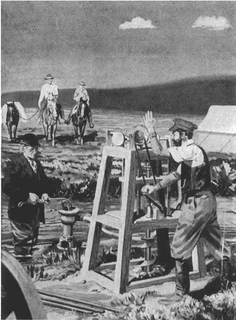
FIGURE C.2 Sweeney’s rotary drill of 1866 had some features in common with rigs of today. Courtesy of NL Baroid.
