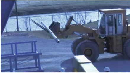
(a) Assembling and carrying the outer tube near the catwalk
