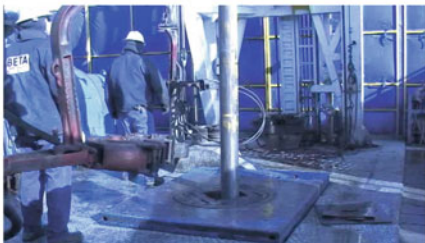
(h) RIH the outer tube assembly
