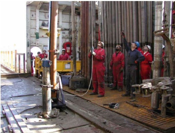
Fig. 14.13 Transferring the LDF from the rig floor to the pipe-deck on the ground (published courtesy of Baker Hughes GE)
