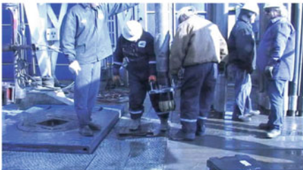
(e) Connect the bit to the stabilizer and the outer tube
