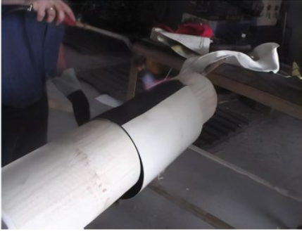
Figure 9.6 (a) Heat shrink sleeve coating on a weld joint in the desert; (b) application.
