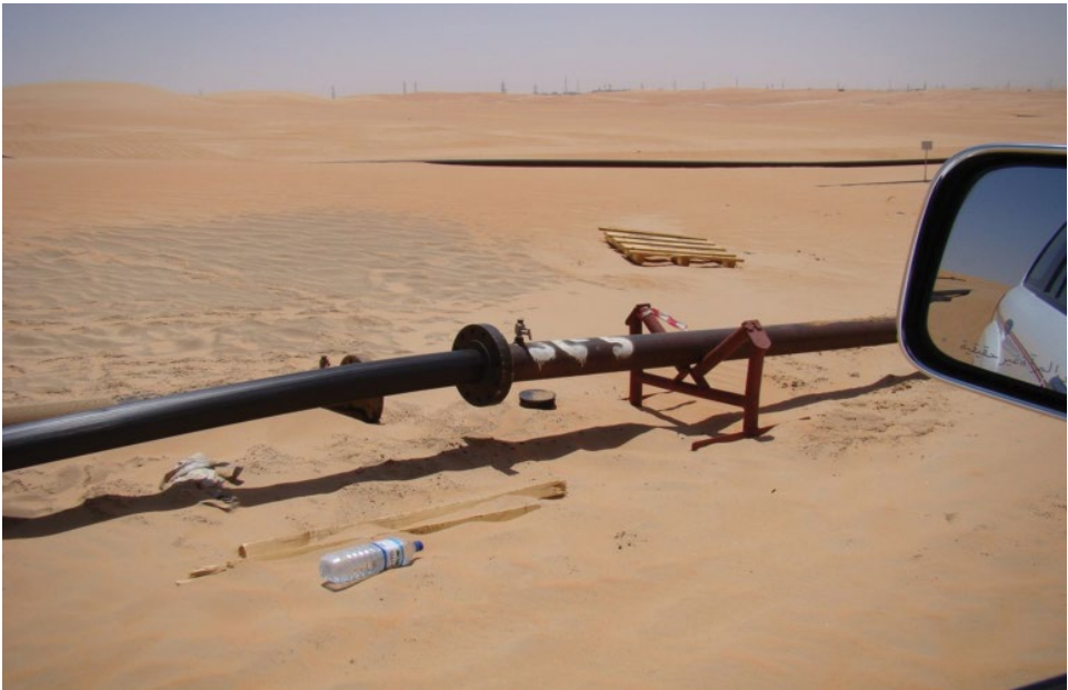
Figure 9.7 Field insertion of HDPE liner in a steel flowline.
