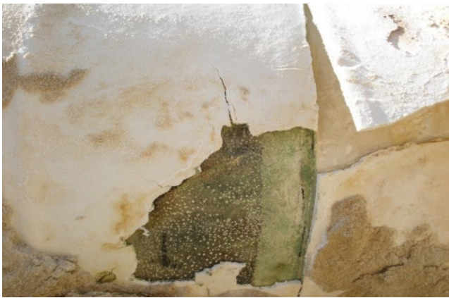
Figure 9.4 Failure of a flame-sprayed PP field joint coating on a three-layer PP-coated gas pipeline. (see colour plate section).
