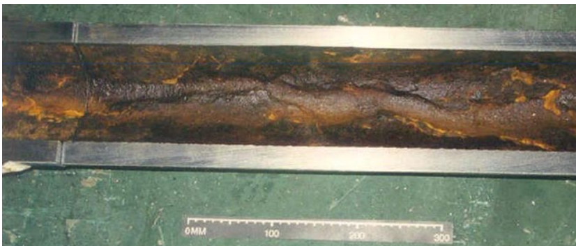
Figure 11.3 Groove corrosion promoted by microbial activity. Source: [2]. (see colour plate section).
