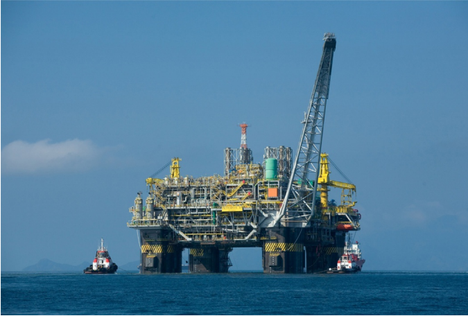
Figure 6.3 Shows a typical semisubmersible platform.
