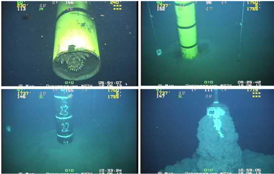
FIG. 13.15 Jetting a conductor in deepwater. Source: Kingdom Drilling training 2014.
