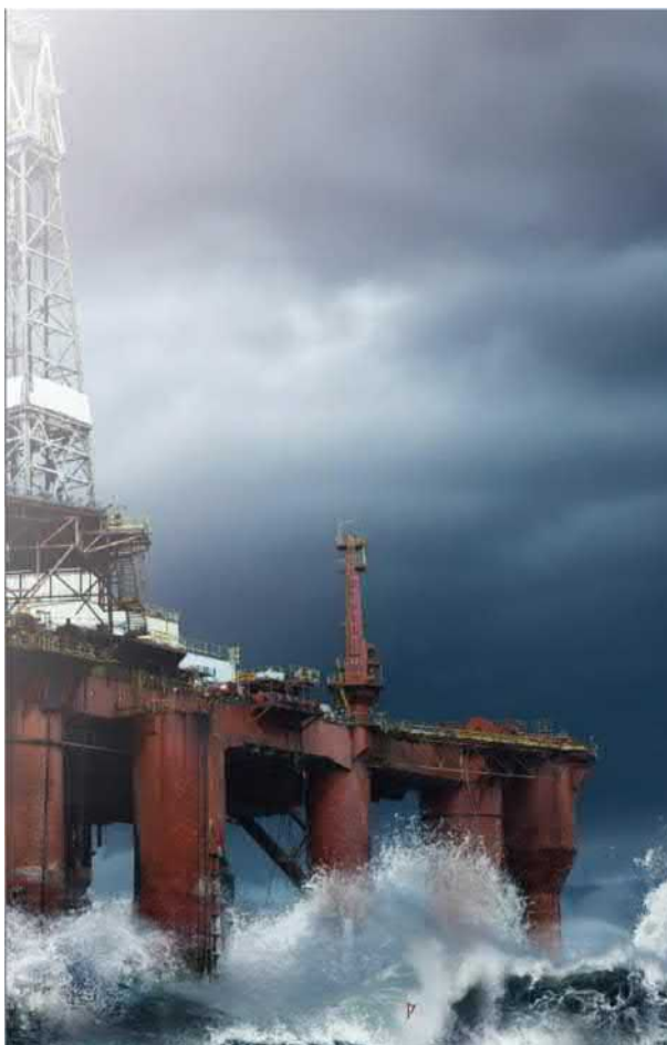
FIG. 4.2 Deepwater rig operating on the Norwegian Continental shelf. Source: Norwegian Deepwater Program 1996–2016.
