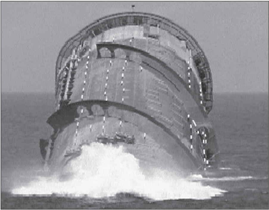
Fig. 9–25. The Genesis spar uprighting from its floating position. (Courtesy Chevron.)
