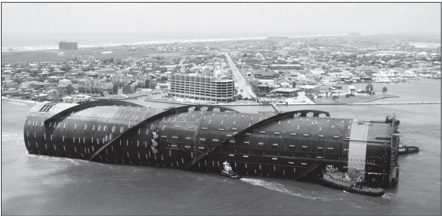
Fig. 9-21. The Genesis spar en route to the well site. Note the spiral strakes. (Courtesy Chevron.)
