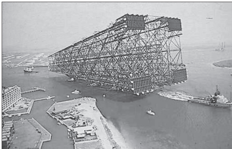
Fig. 1-16. The Bullwinkle Platform being towed to sea. (Courtesy Shell International, Ltd.)
