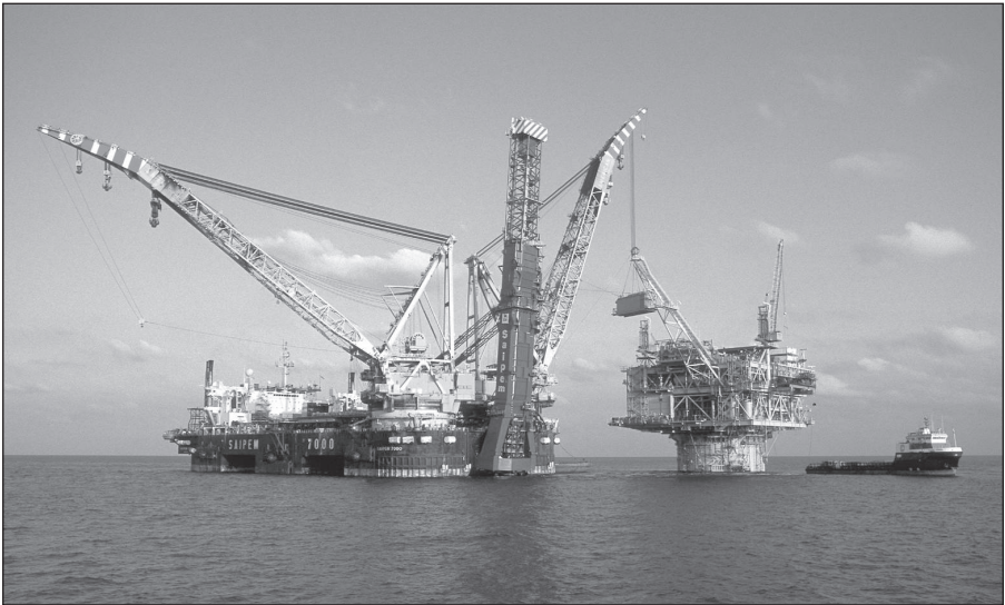
Fig. 8–15. Saipem 7000 heavy-lift crane vessel setting a deck. (Courtesy Saipem.)
