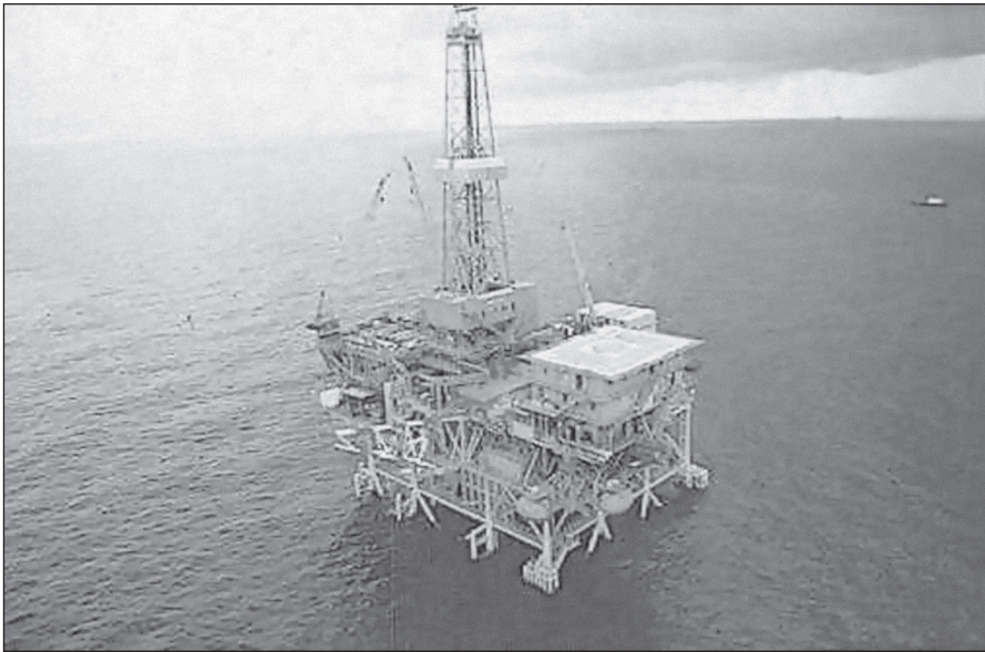
Fig. 1–17. The Bullwinkle Platform in place. (Courtesy Shell International, Ltd.)
