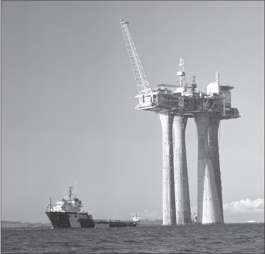
Fig. 8–9. Concrete gravity structure Troll being towed to its North Sea installation site. (Courtesy Norske Shell.)
