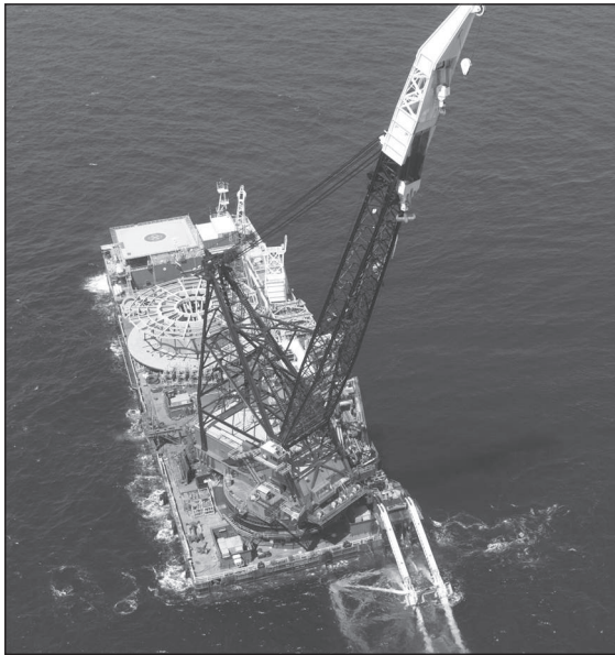
Fig. 12-11. Reel barge Hercules laying pipe. (Courtesy Global Industries.)
