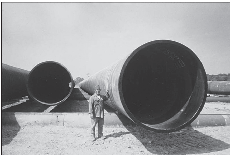
Fig. 8-7. A 96-inch diameter steel pile in fabrication yard
