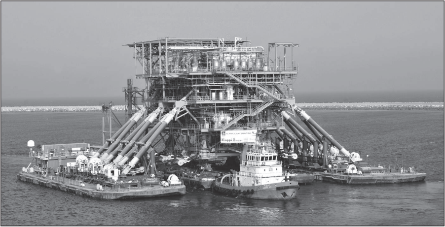
Fig. 9-8. A truss lift system that floats over a platform to set a topsides. (Courtesy Versabar.)
