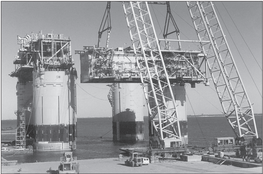
Fig. 11-7. Deck module being lifted onto the Mars TLP. (Courtesy Shell E&P)
