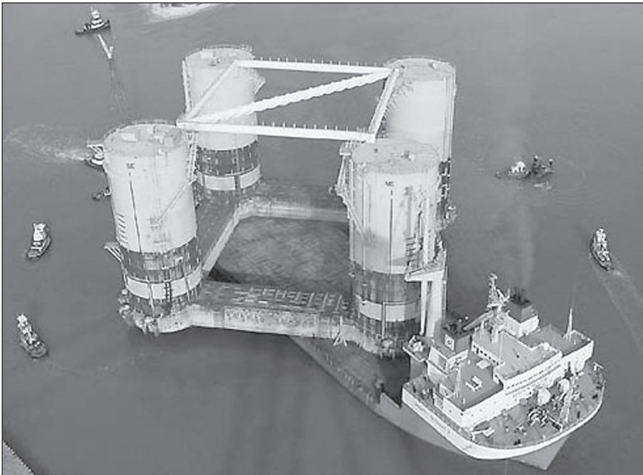
Fig. 13–4. Hull of TLP Brutus en route to installation on a heavy lift vessel. (Courtesy of Dockwise USA.)
