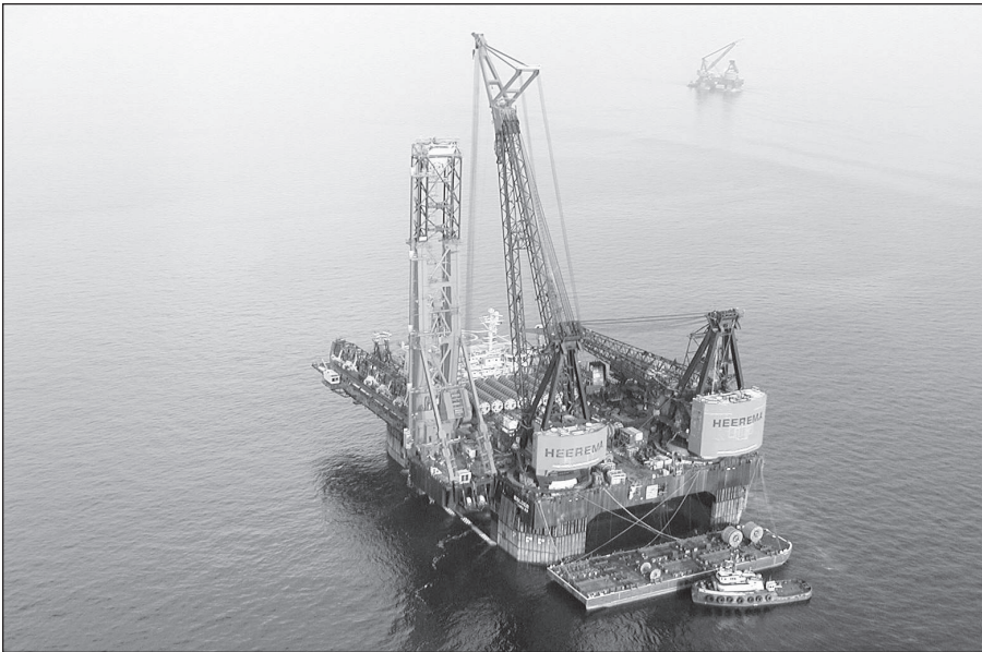
Fig. 12–7. J-lay tower on the crane vessel Balder . (Courtesy Heerema Marine Contractors.)
