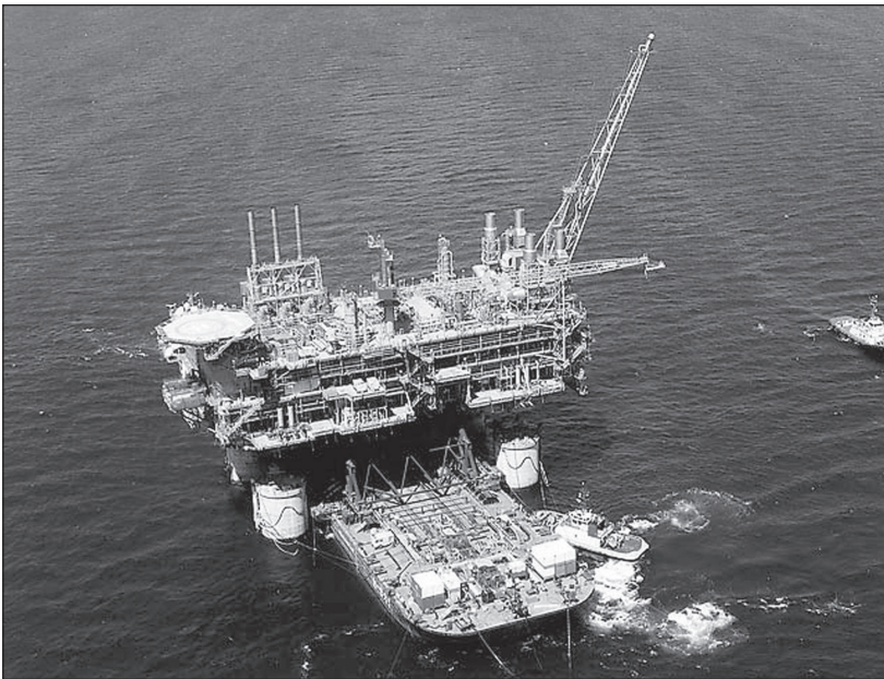
Fig. 8–16. Malampaya deck being floated in to be lowered onto the structure legs. (Courtesy Philippines Exploration BV.)
