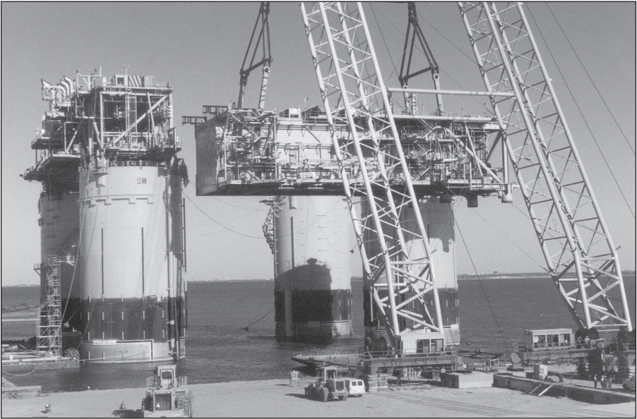
Fig. 9-9. Integrating topsides with hull using an onshore special lifting device. (Courtesy Shell E&P)
