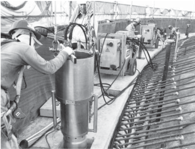
Fig. 8.22 Stressing the vertical strands.
