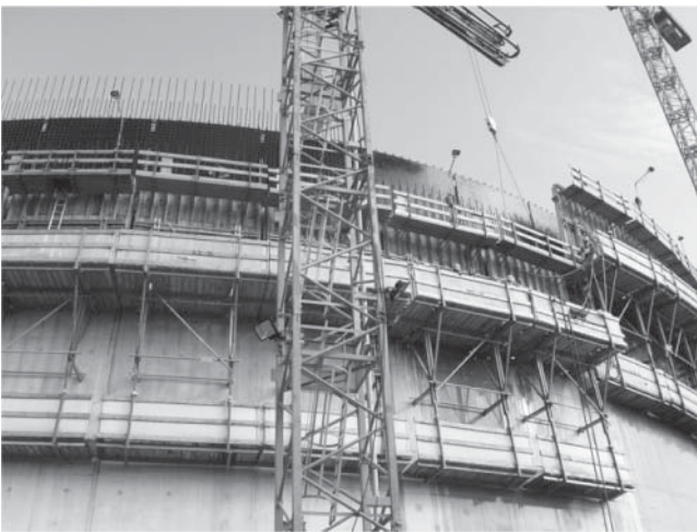
Fig. 8.11 Climbing formwork being repositioned for next lift.
