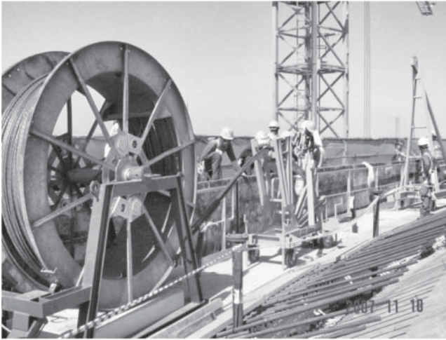
Fig. 8.21 Installing vertical tendons.
