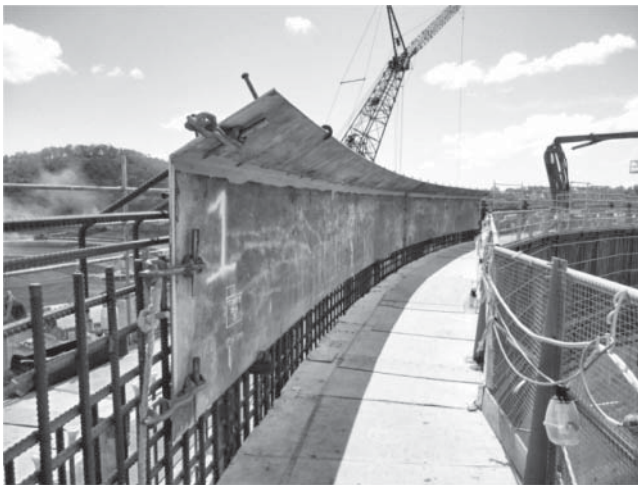
Fig. 8.3 Installing the compression ring.
