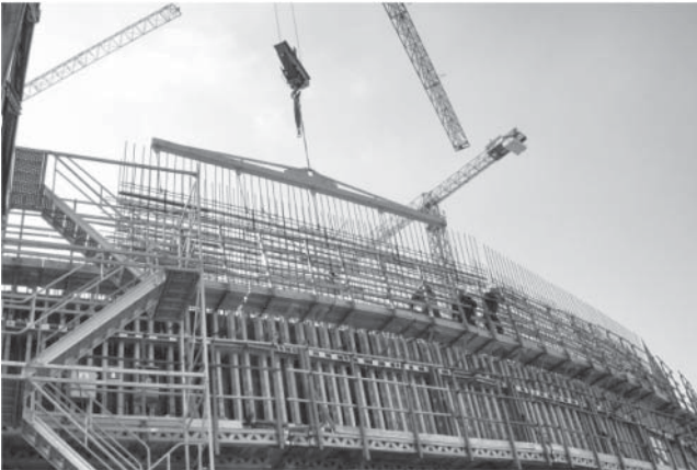
Fig. 8.16 Large reinforcement mesh suspended from a crane spreader beam.
