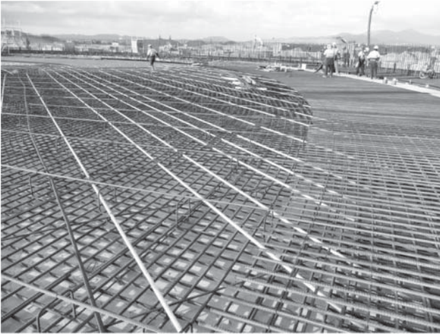
Fig. 8.24 Cable conduits for heating cables in middle of base slab.
