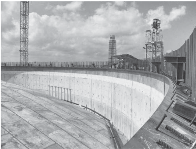
Fig. 8.6 “Roof air raising”.
