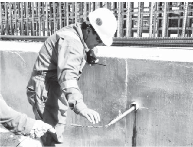
Fig. 8.27 Taking inclinometer readings.
