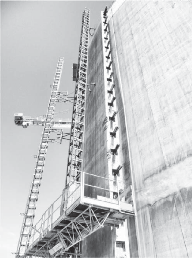
Fig. 8.23 Working platform for horizontal stressing.
