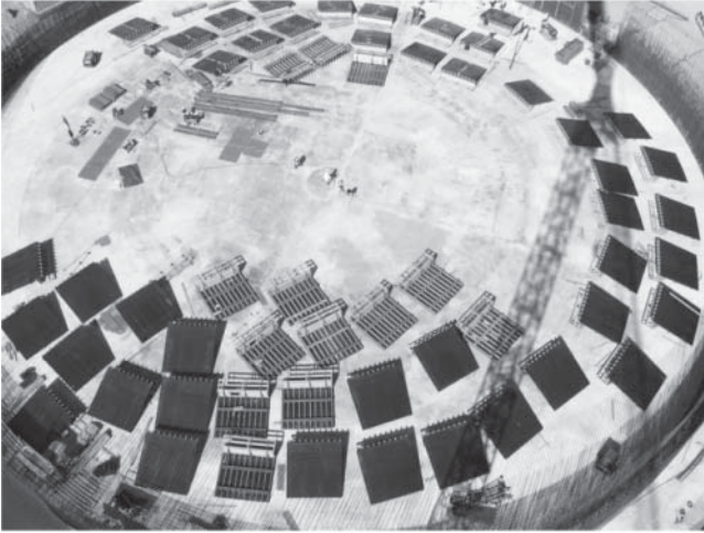
Fig. 8.10 Preparing the wall formwork elements.
