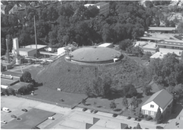
Fig. 2.4 Peak-shaving plant in Stuttgart, Germany.
