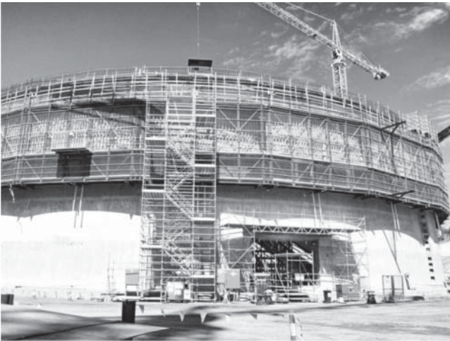
Fig. 8.8 Temporary opening.
