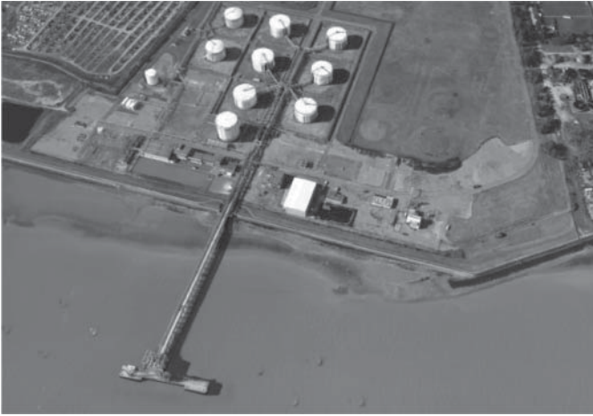
Fig. 2.3 Canvey Island receiving terminal.
