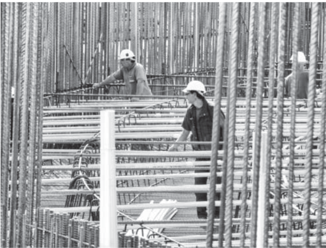
Fig. 8.25 Laying cable conduits for heating cables around the perimeter.
