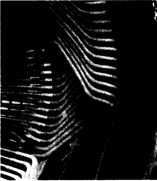
Figure 3.28 A double-layer 11 kV diamond winding in progress, with two bracing rings (Courtesy: Laurence, Scott Electromotors Ltd.)
