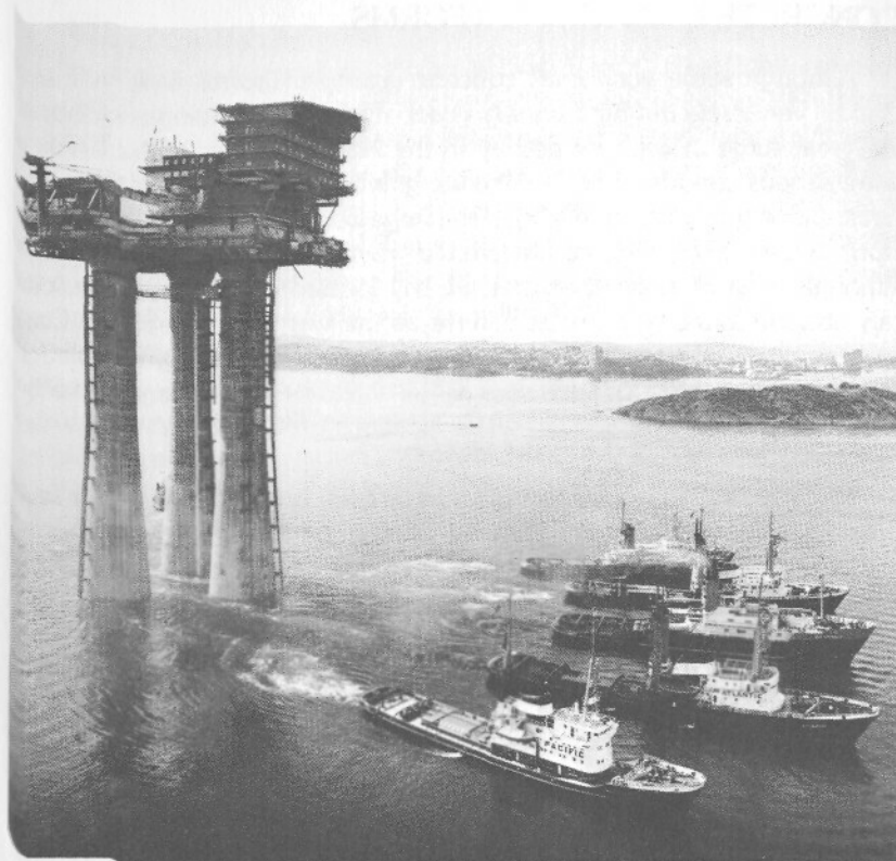
FIG. 1-6 Towing the concrete gravity platform to the installation site.
