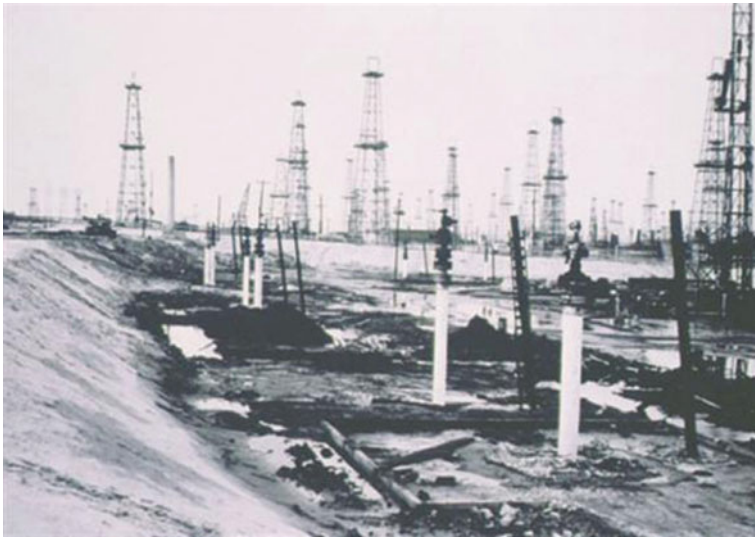
Picture 11.1 Ground subsidence can be tangibly ‘felt’ in shallow reservoirs that produce oil and sand.
