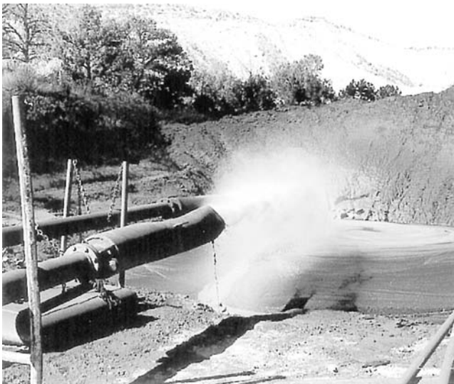
Figure 19.7. Foam at the flowline.
