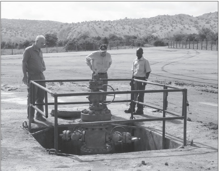
Fig. 3–9. Wellhead inside cellar after rig departed
