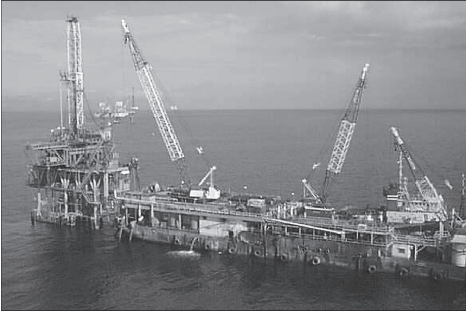
Fig. 5-7. Drilling tender with derrick on platform
