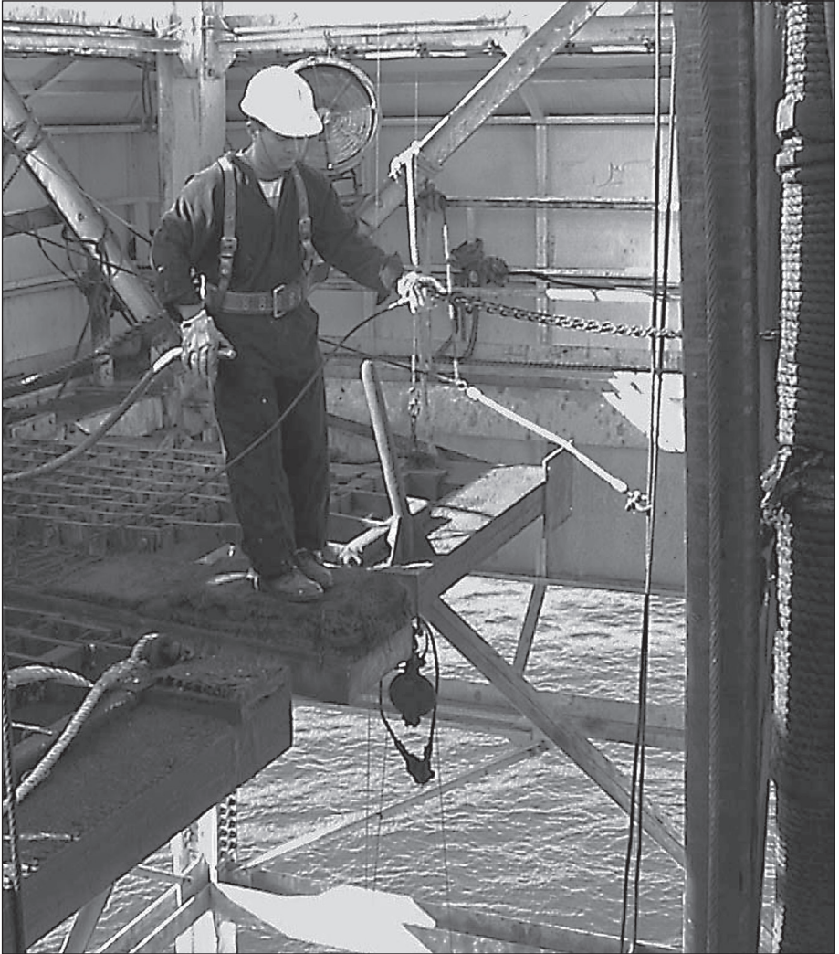
Fig. 14–4. Man working high in the derrick (note the safety harness)
