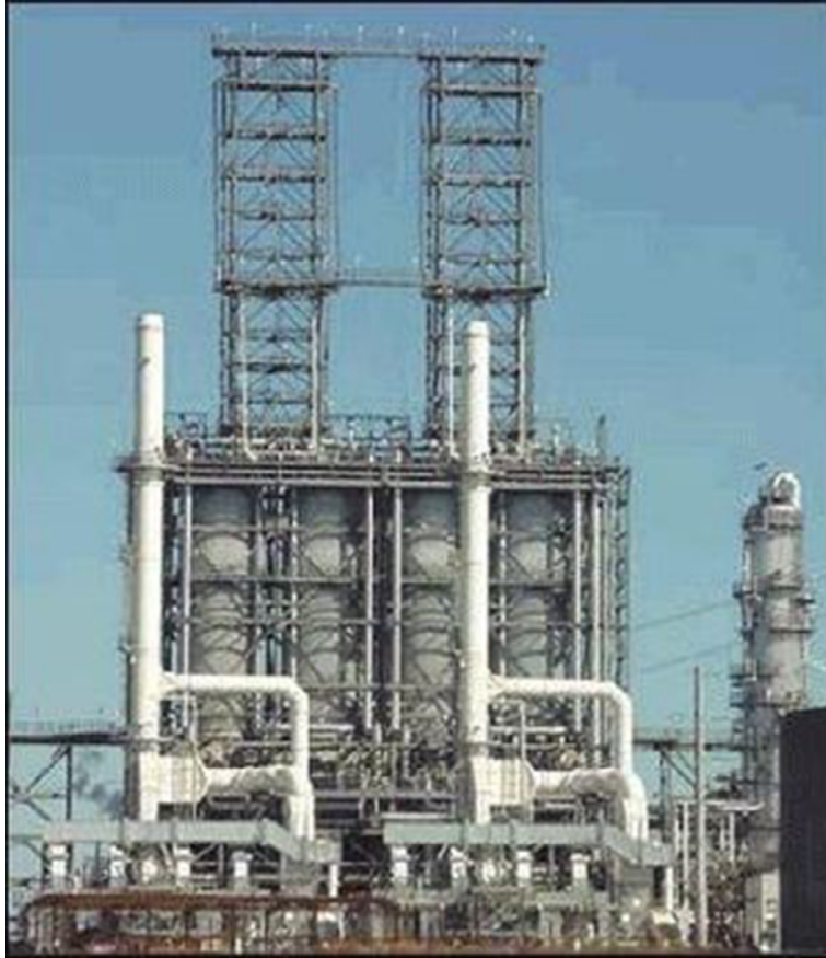
Photo of a coker unit drill structure
