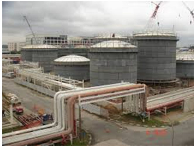
Photo of coned roof storage tanks
