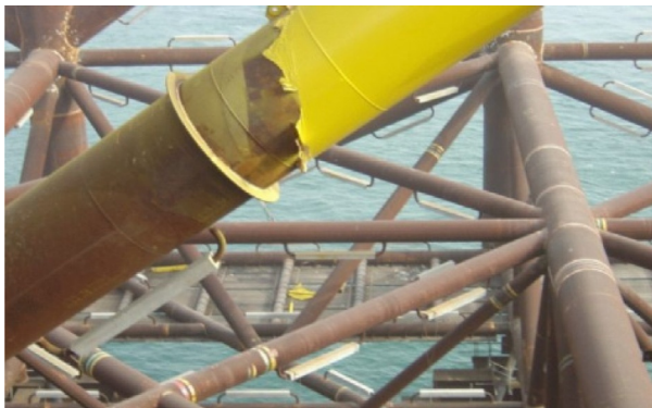
Sacrificial anodes on an offshore jacket
