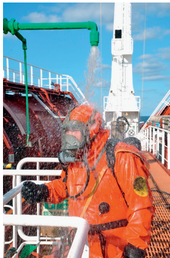
Eyewash and Safety Shower
