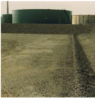
Photo of earth dike
