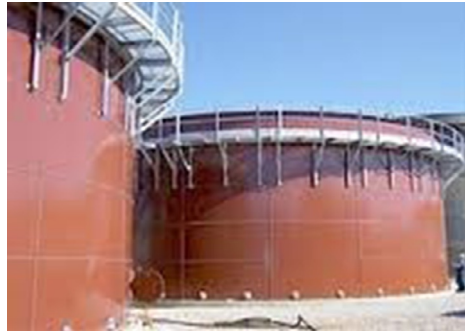
Top platform outside tank wall
