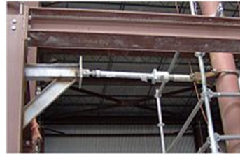
Photo of snubber in a plant
