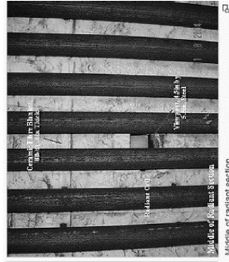
RADIANT TUBE REMOVAL IN A CIRCULAR FURNACE
