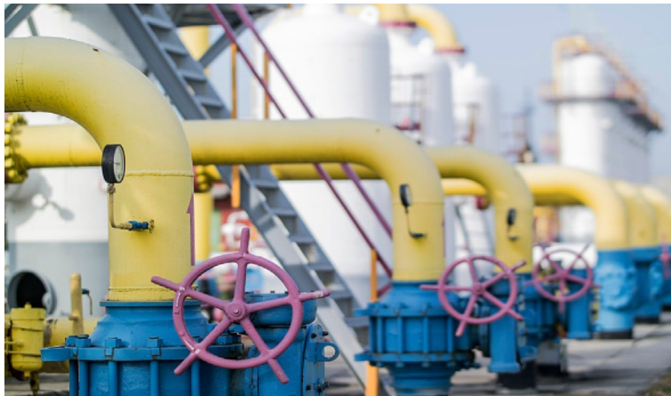
Photo showing pressure gauges
