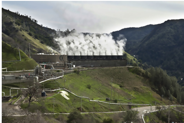
FIGURE 7.3 The Geysers geothermal power plant in California. California State Energy Commission photograph.
