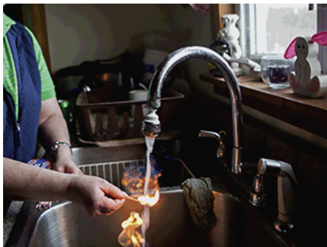
FIGURE 6.1 A flammable kitchen faucet caused by natural gas entering a water supply well in Pennsylvania. Some people have linked this to fracking. Photo copyright Getty Images, used under license.
