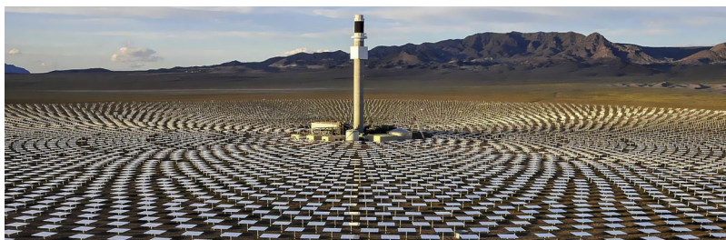
FIGURE 7.4 Crescent Dunes solar power tower surrounded by 10,347 heliostat mirrors in the Nevada desert near Tonopah. Photo from DOE, National Renewable Energy Laboratory.
