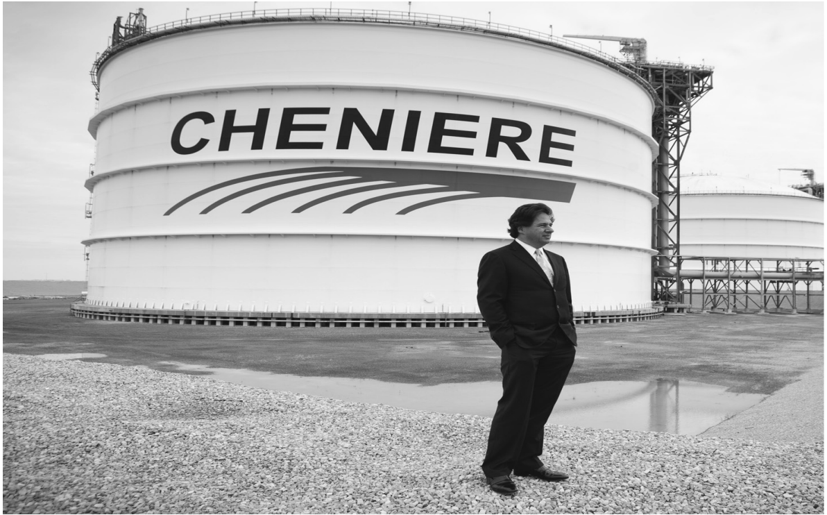
Charif Souki at his company's Louisiana LNG terminal.
