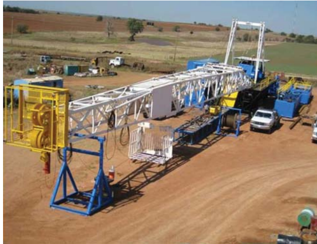
Fig. 1.11 —Rig with cantilever derrick (Derrick Engineering Company 2010).
