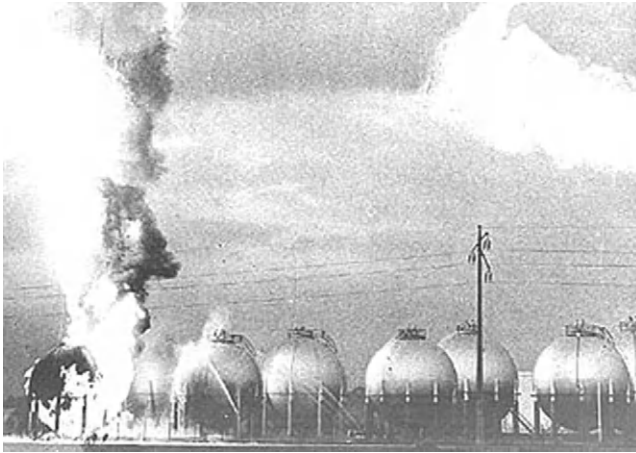
FIGURE 5-9 BLEVE in LPG sphere, Feyzin, France, 1966 (LPG sphere pre-accident). (Source: http://www.musee-pompiers.asso.fr/images/cs-dat-01.jpg .)
