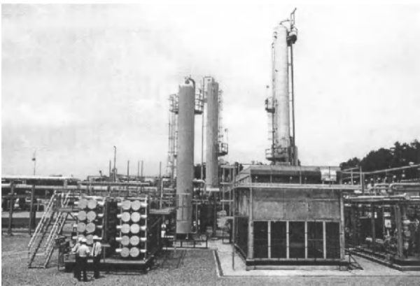
FIGURE 1-27 Size comparison of membrane and amine systems.
