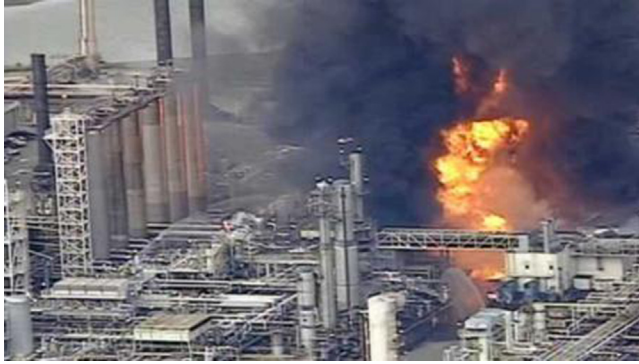
Figure 6.5 Richmond, California refinery incident, 2012.
