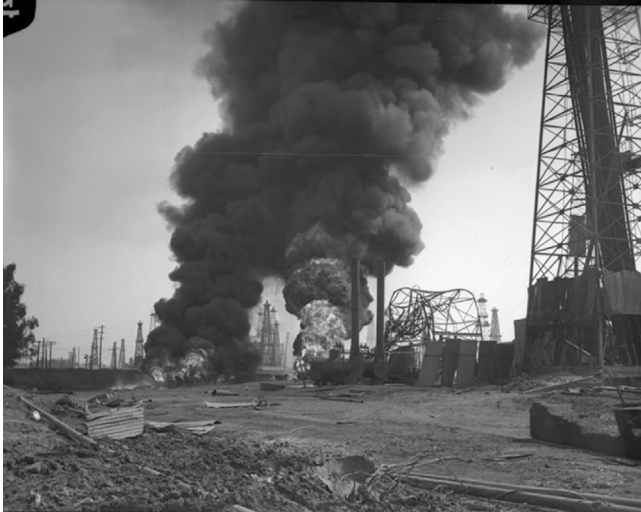
Figure 1.2 Early petroleum industry fire incident.
