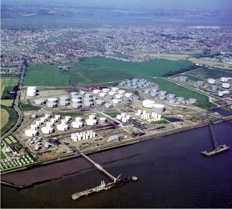
Figure 8.2 Tank farm segregation.
