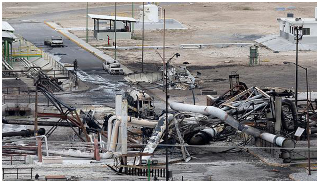
Figure 6.4 Reynosa, Tamaulipas Mexico, gas plant explosion and fire.
