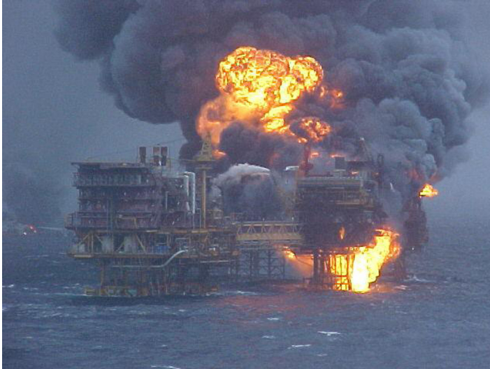
Figure 6.11 Offshore platform fire incident, Indian Ocean, 2005.
