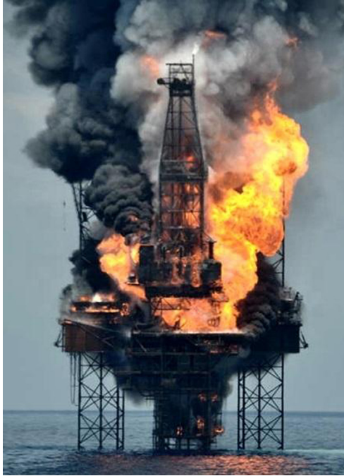
Figure 6.9 Montara oil field, Australia, offshore oil production, explosion and fire.
