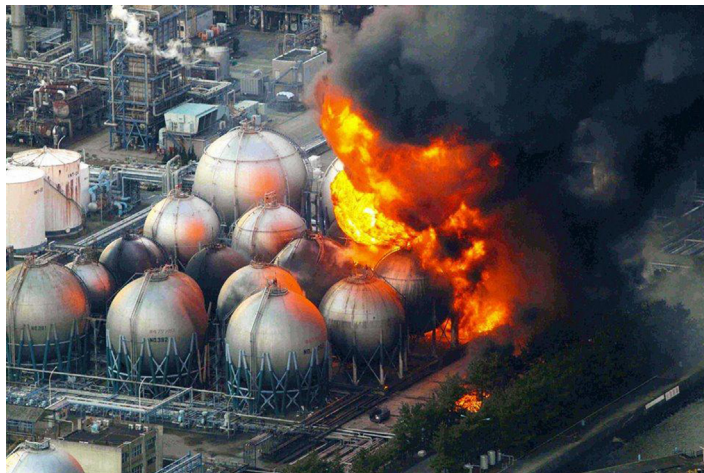
Figure 6.6 Earthquake impact, refinery fire, Canada 2011.
