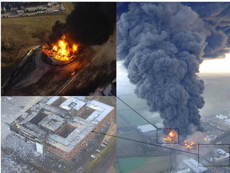
Figure 6.10 Buncefield oil depot incident.
