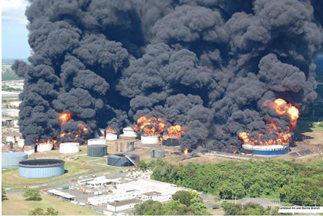
Figure 6.8 Storage tanks burning as pool fires, Puerto Rico, 2009. Photo Credit CSB.
