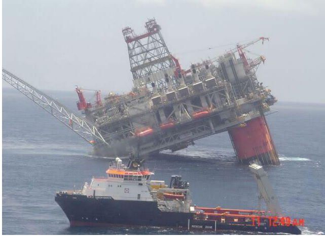
Figure 7.3 Lack of adequate buoyancy for semisubmersible platform.
