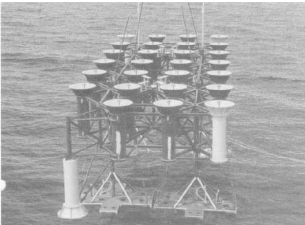
Figure 14.20 Subsea template lifting
