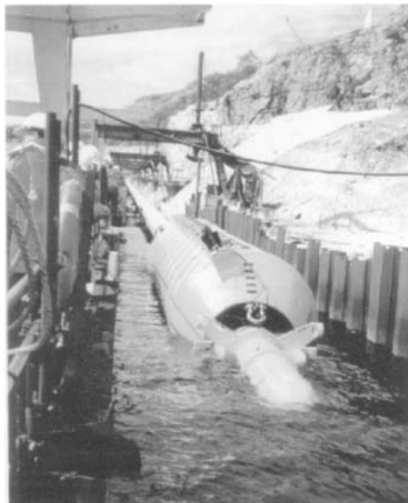
Figure 14.9 Buoyancy modules fitted to the Heidrun TLP tendons
