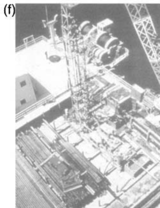
Figure 16.20 Examples of geotechnical drillings (Continued)
