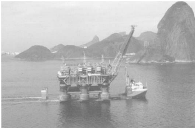
Figure 14.24 Dry transport of P-40 on self-propelled vessel mighty servant 1
