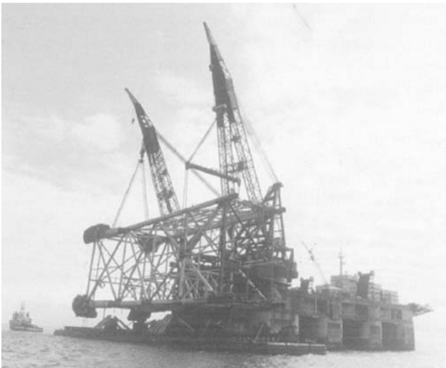
Figure 14.1 Two block upending (Marathon East Brae jacket)
