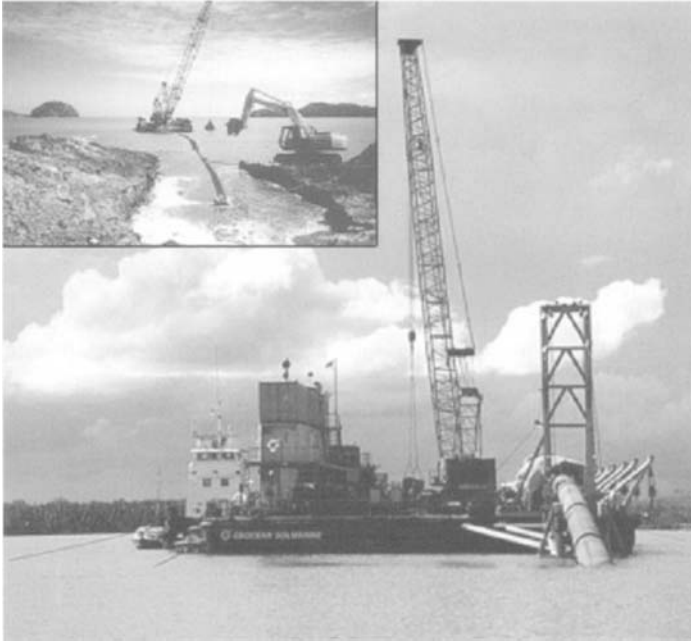
Figure 14.30 Shore pull operation
