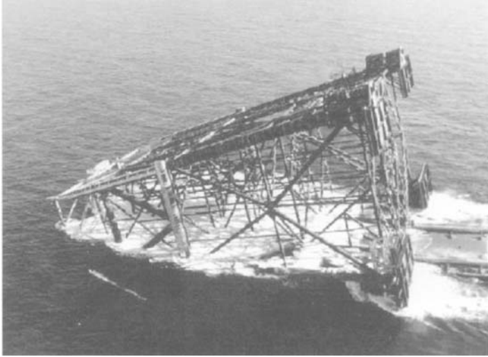
Figure 14.27 Launching of a 4-Leg Jacket
