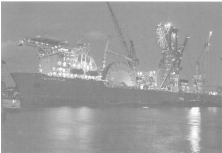
Figure 14.31 Deep Blue reel pipelay vessel
