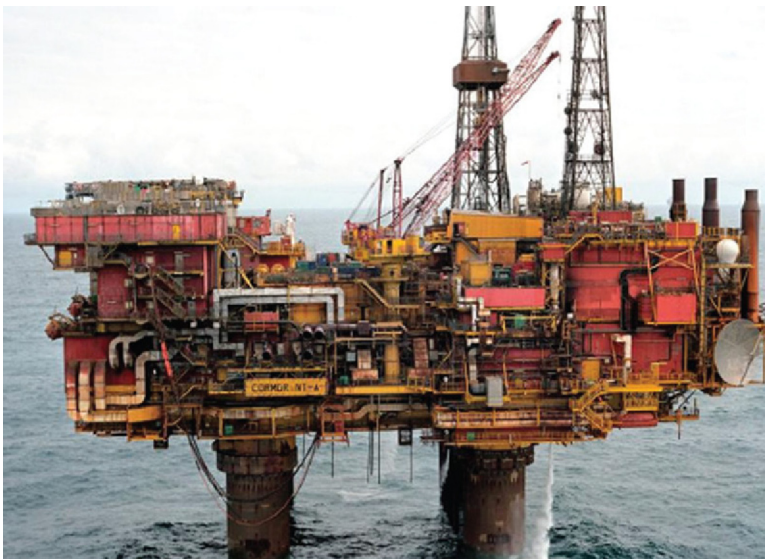
Figure 3.2 Concrete gravity platform.
