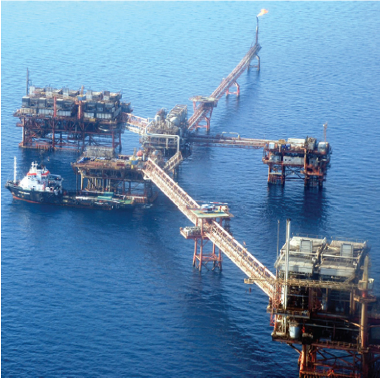
Figure 6.2 Production and drilling complex. Source: Figure reproduced from El-Reedy, 2012, fig. 1.7.
