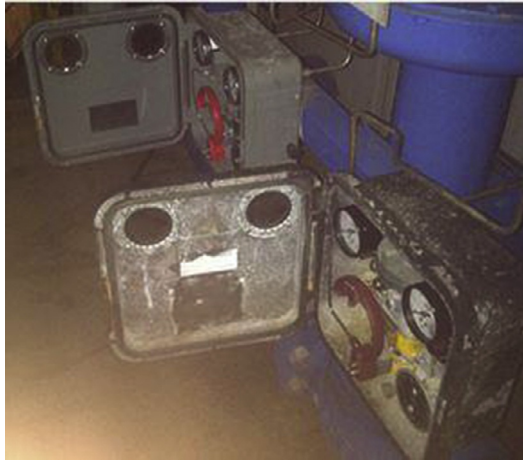
Fig. 12.8 Liquid level controller (LLC).
