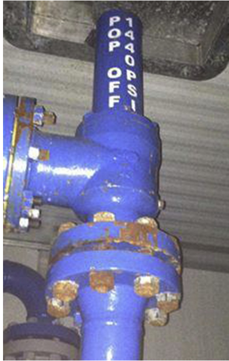
Fig. 12.10 Mechanical pop-off.
