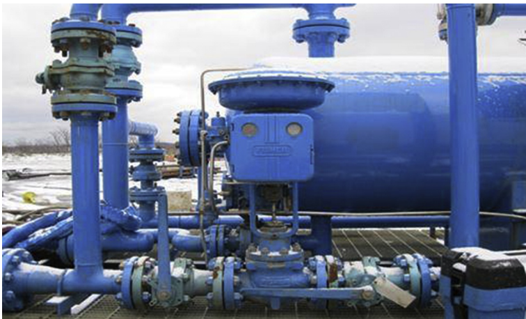
Fig. 12.9 Back pressure regulator (BPR).
