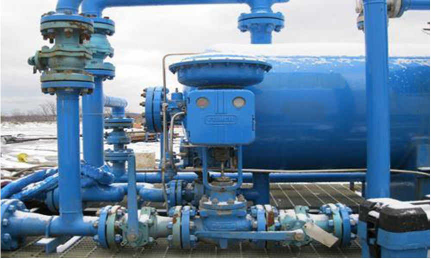
Figure 12.9 Back pressure regulator (BPR).
