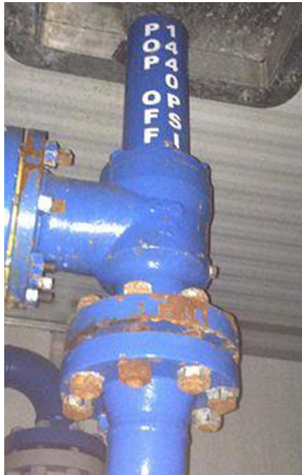
Figure 12.10 Mechanical pop-off.
