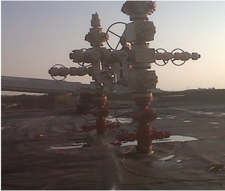
Figure 16.28 Typical frac wellhead.
