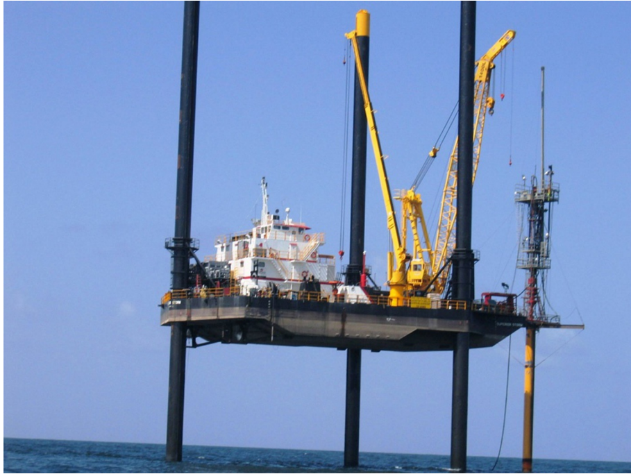
■ FIG. 5.17 Lift boat and outriggers. (Courtesy of International Snubbing Services.)
