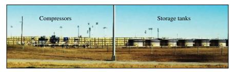
FIGURE 14.11 Surface equipment at a shale gas well pad.
