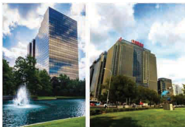
Figure 13.1. Sinopec headquarters, Houston and Beijing.
