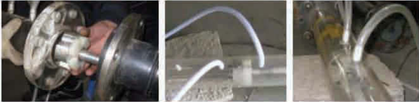
Figure 1.5h. Siren test sections with differential transducers for signal strength measurement (not influenced by reflections and propagating noise).
