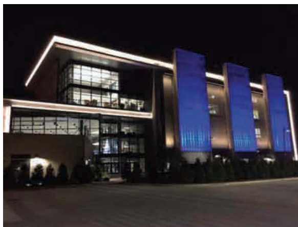
Figure 15.1. Oil and Gas Technology Center (Oklahoma City).
