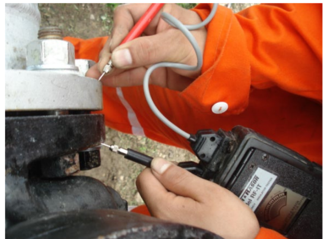
Figure 5.14 Continuity testing to be sure that electrical isolation has been achieved.
