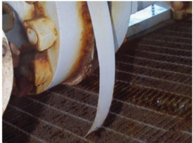
Figure 5.49 Pack rust on a flange causing the flange protector to distort (a) and eventually break (b). Source: Reproduced with permission from Deepwater Corrosion Services Inc. [56].
