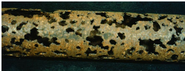
Figure 8.17 Corroded downhole tubing caused by leaving acid treatment in tubing for too long.
