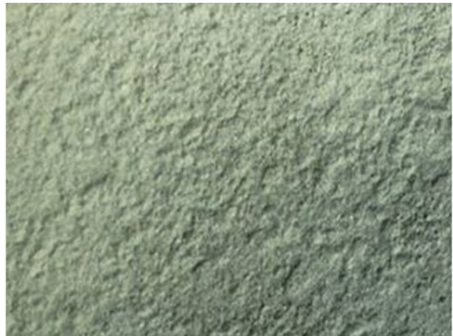
Figure 6.5 The surface of a pipeline ready for recoating in the field.
