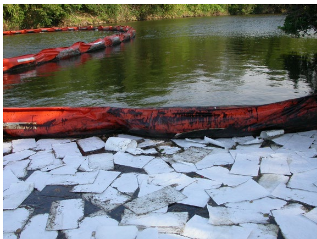
Figure 1.3 An oil containment boom to minimize the spread of crude oil from an external corrosion leak on a submerged pipeline.
