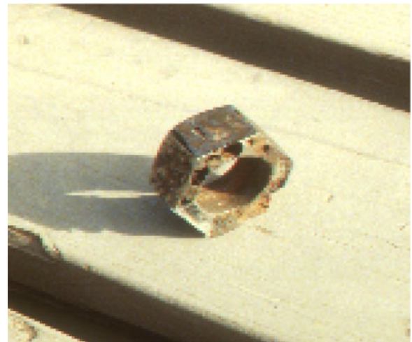
Figure 5.60 Intergranular corrosion along the forming direction on a stainless steel nut.
