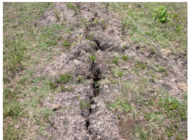
Figure 3.12 Cracked soil due to drying after the rainy season.
