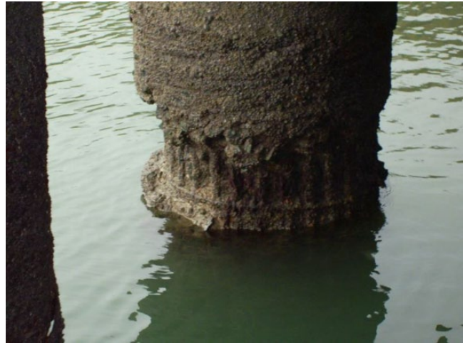
Figure 3.10 Waterline corrosion.
