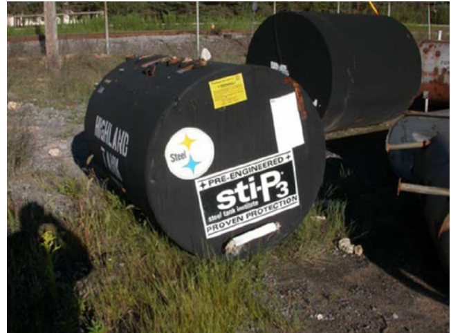
Figure 6.101 STI P3 tanks in storage prior to installation.
