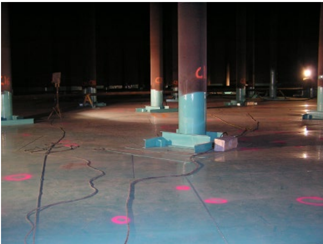
Figure 8.49 Painting for corrosion control on the lower portions of vertical supports on a large AST.
