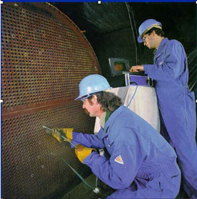
Figure 7.17 Eddy current inspection of heat exchanger tubes. Source: From Ref. [3].
