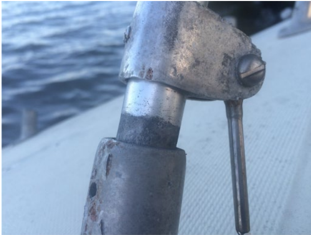
Figure 5.53 Crevice corrosion of aluminum shaft beneath a fitting.
