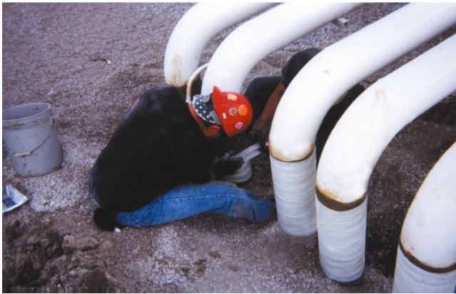
Figure 6.28 Petrolatum tape with glass-reinforced outer wrap used at the air-soil interface on piping. Source: Photo courtesy Denso North America Inc.
