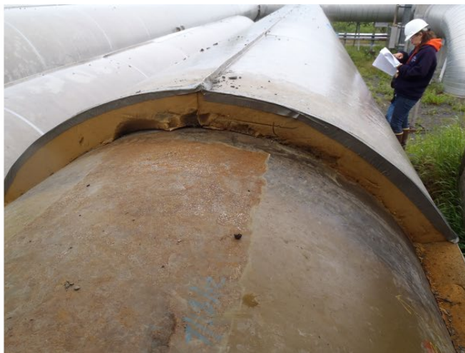
Figure 8.66 Voids in insulation.
