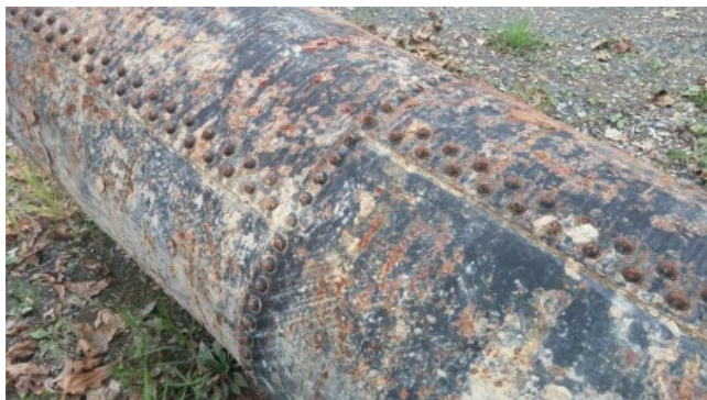
Figure 4.45 Riveted carbon steel water pipeline that remained in service for over 100 years. Source: Photo courtesy K. Rickvalsky, McWayne Ductile, www.mcwaneductile.com.
