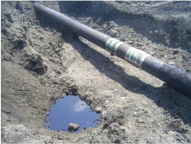
Figure 8.88 Repair sleeves installed on corroded crude oil pipeline.
