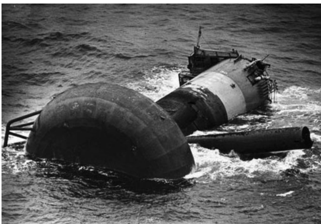
Figure 8.108 The capsized Alexander Kielland floating offshore platform.
