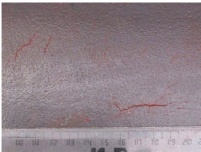
Figure 7.8 Magnetic particle crack indications on the exterior of a petroleum pipeline.
