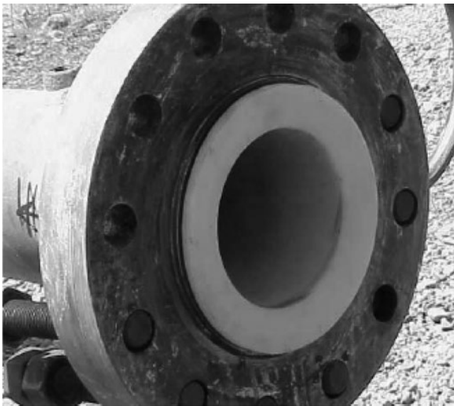
Figure 6.24 The flange end of a liner segment installed in an oilfield pipeline.
