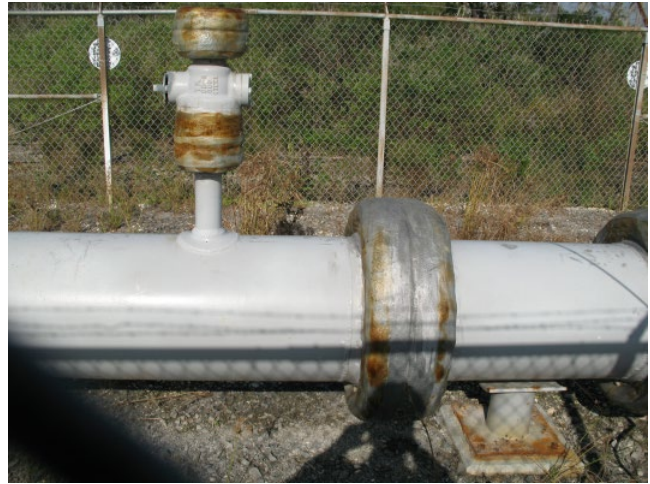
Figure 6.29 Reinforced wraps used to coat flanges on above-ground piping systems.
