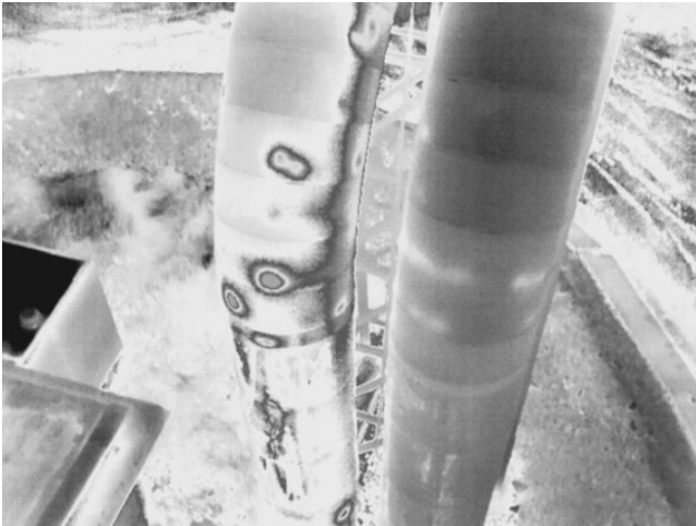
Figure 7.21 Thermal imaging of piping on an offshore platform. http://diydrones.com/profiles/blogs/pipeline-inspection-with-uav-thermal-diagnostics , 28 February 2017.
