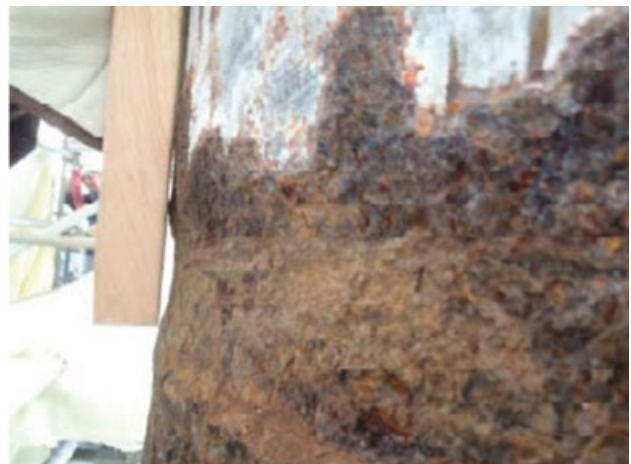
Figure 8.73 CUI on vertical piping near the locations shown in Figure 7.23a and b where obvious moisture problems could have been noted and reported.
