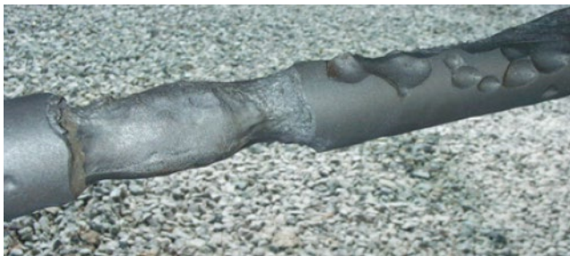
Figure 5.118 Stray current corrosion of a stainless steel propeller shaft. Source: Photo courtesy of Dudley Gibbs, Dudley's Marine Electric, Humacao, Puerto Rico, USA.
