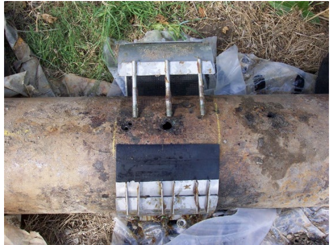
Figure 8.87 Installation of a pipeline repair sleeve over a corroded pipeline leak.
