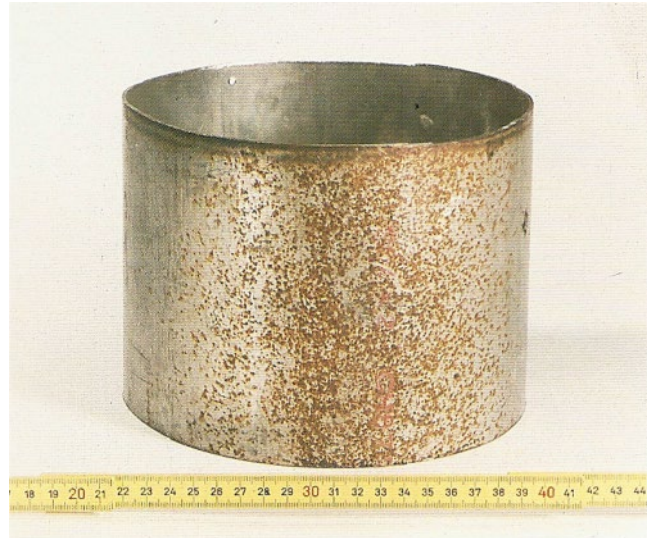
Figure 5.110 Contact corrosion on stainless steel piping caused by grinding debris from nearby carbon steel. Source: Bogaerts [82]. Reproduced with permission of NACE International.
