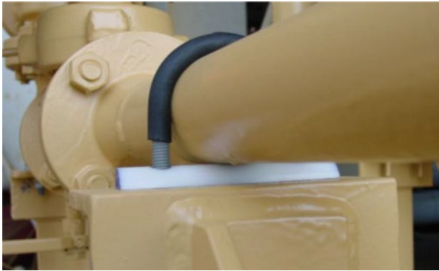
Figure 5.48 Commercially available pipe restraint intended to minimize CUPS. Source: Reproduced with permission from Deepwater Corrosion Services Inc. [56].
