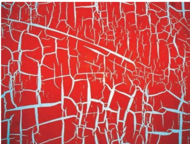
Figure 6.40 Alligatoring of a protective coating [69, 70]. Source: Reproduced with kind permission of Brendan Fitzsimons, FITZ-COATINGS Ltd.
