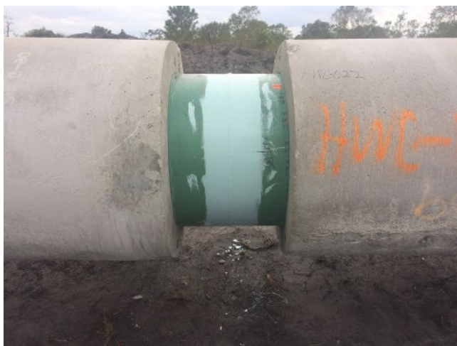
Figure 8.104 Field-applied protective coating at girth weld location between two weight-coated joints.
