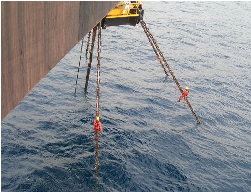
FIGURE 12.4 Rope-access specialists climbing down to inspect chain in splash zone.
