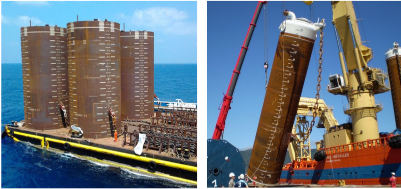
FIGURE 8.2 Suction piles. Courtesy: SPT Offshore.
