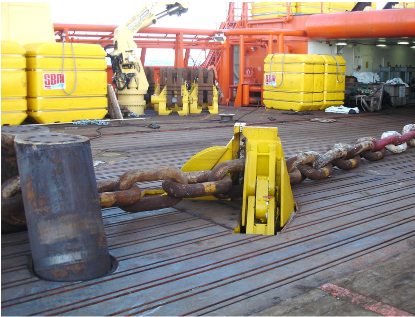
FIGURE 11.7 Chain gets pulled through the towing pins (left) on the deck and secured by the shark jaws (middle).
