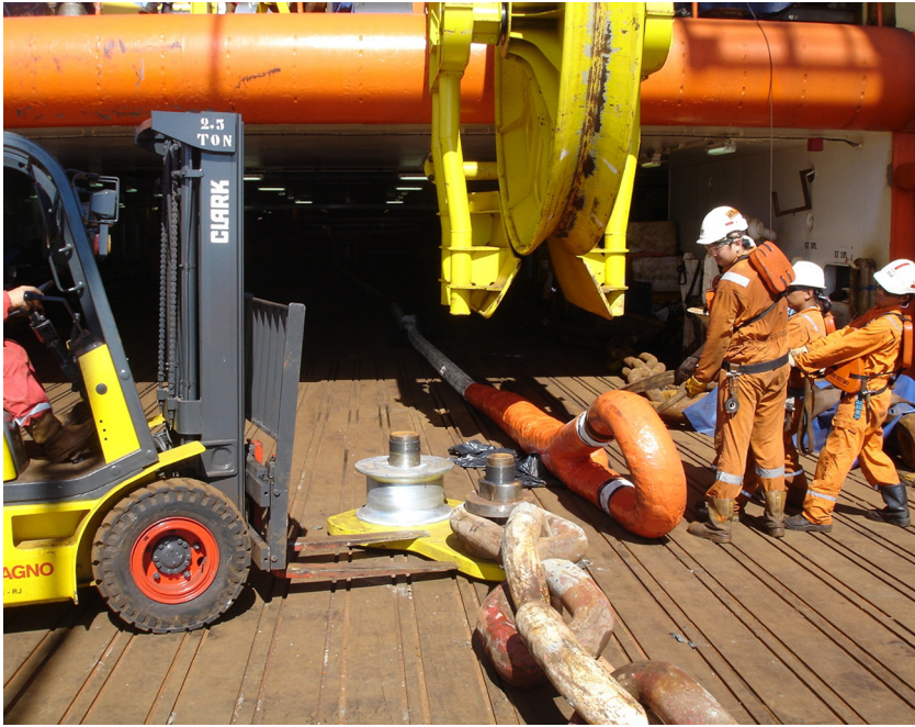
FIGURE 11.5 Connecting polyester rope with an H-link to bottom chain.
