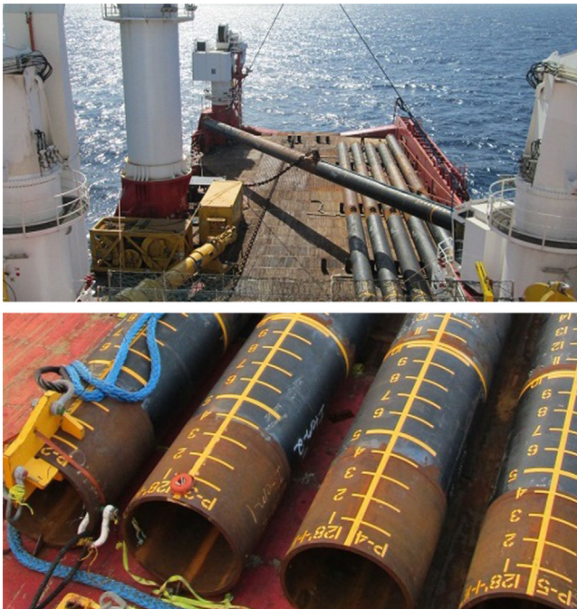
FIGURE 8.4 Driven piles. Courtesy: InterMoor.
