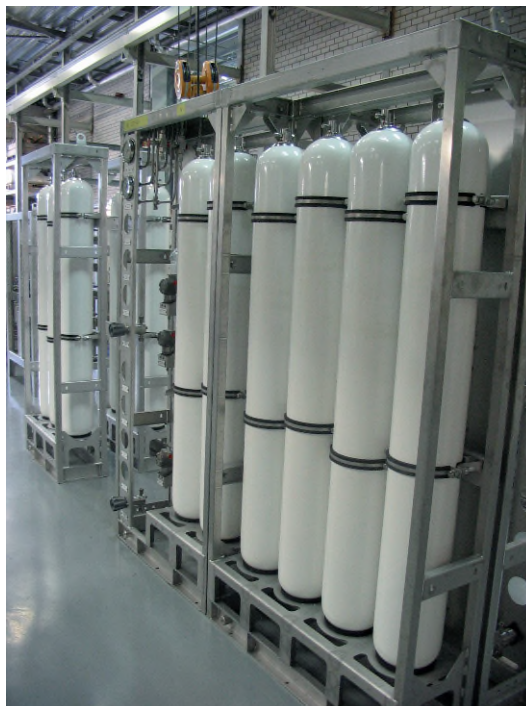
Fig 11.7.C A number of accumulators in parallel might be necessary to provide the storage of hydraulic power. (Courtesy of Frames)
