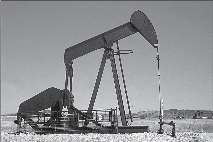
Plate 19-7. Artificial lift with a sucker-rod pumping unit
