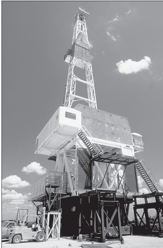
Plate 15-1. Rotary drilling rig. (Courtesy of Parker Drilling.)
