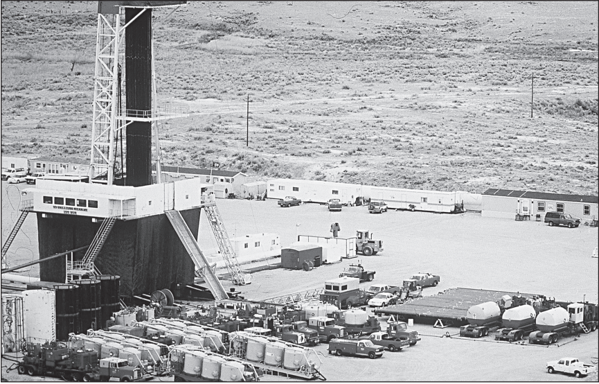
Plate 19-4. Cement job. (Courtesy of Halliburton.)
