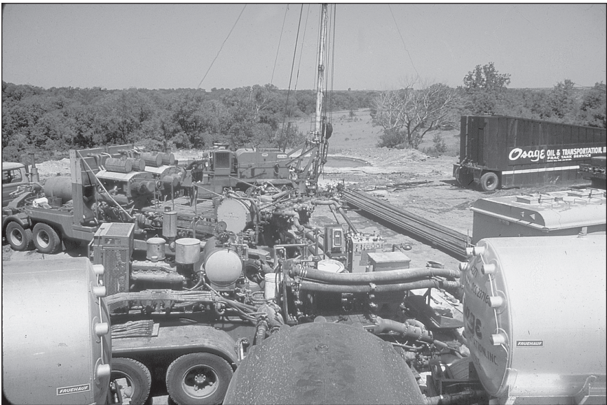
Plate 24-1. Hydraulic fracturing an oil well
