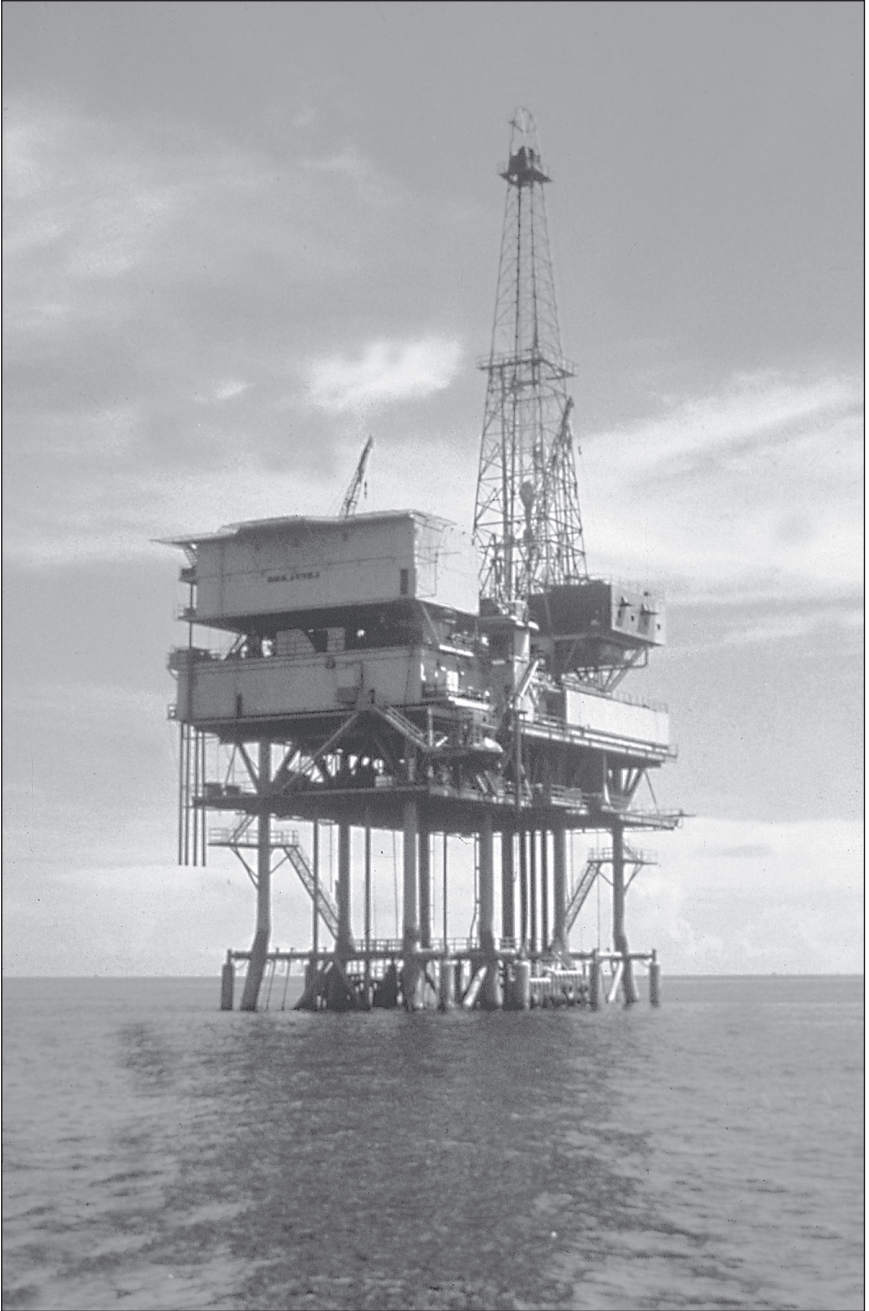
Plate 21-1. Fixed production platform. (Courtesy of American Petroleum Institute.)
