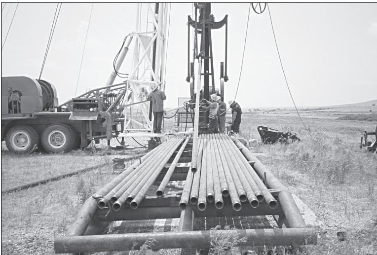
Plate 19-5. Tubing being run into a well
