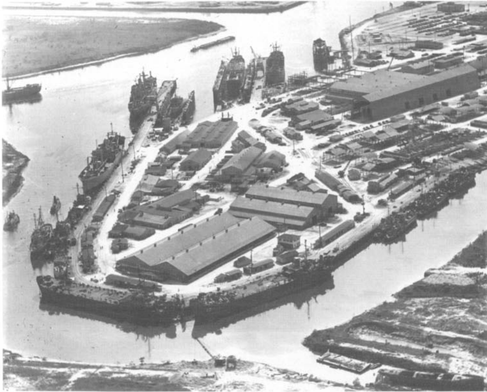
Brown Shipbuilding—Greens Bayou during World War II
