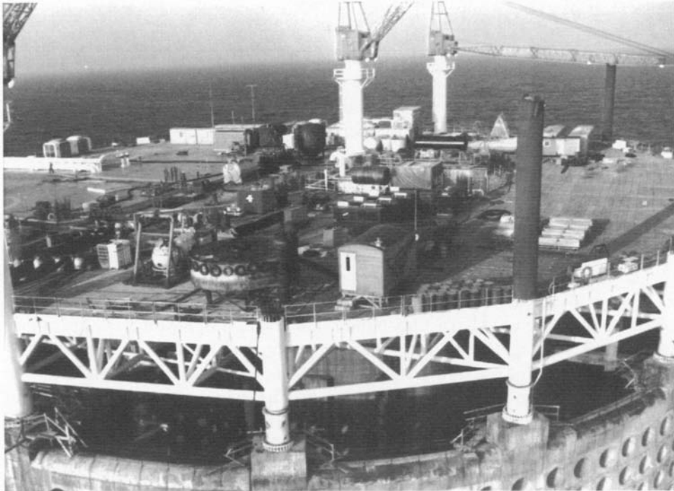
Ekofisk concrete tank. Photo courtesy of Dirk Blanken
