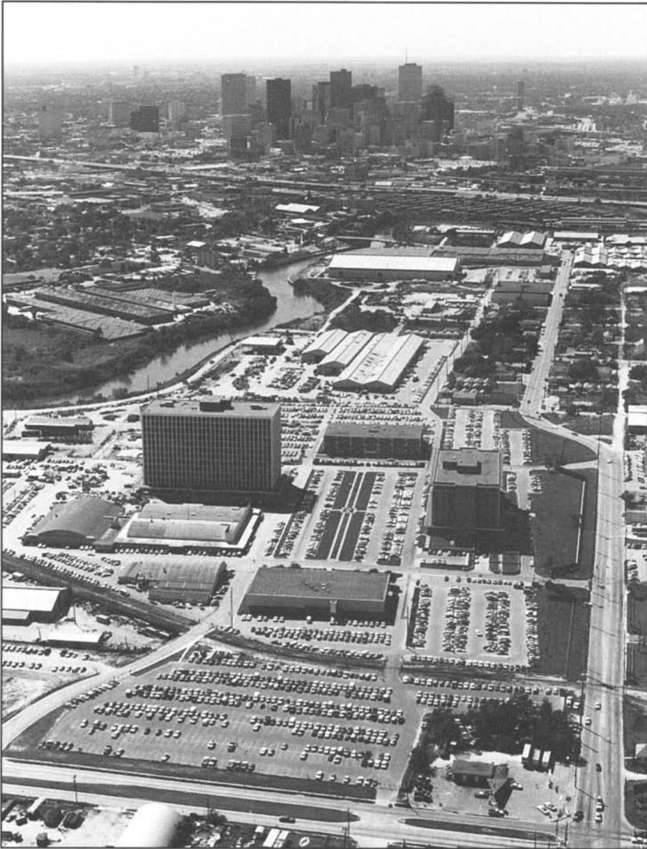
Offices on Clinton Drive, Houston
