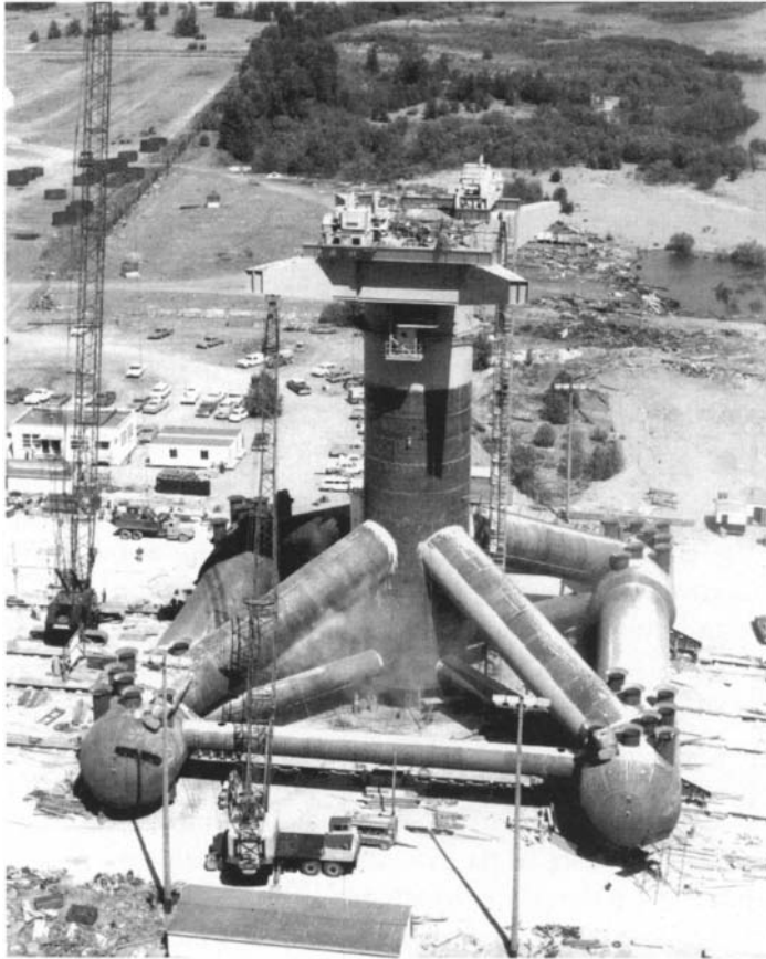
Monopod under construction
