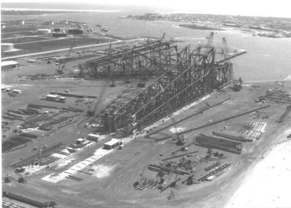
Fabrication of Chevron’s Garden Banks jacket at Harbor Island
