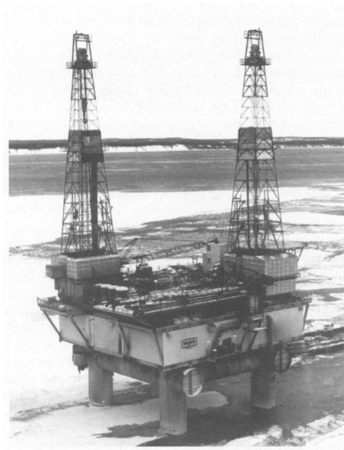
Four-legged platform in Cook Inlet
