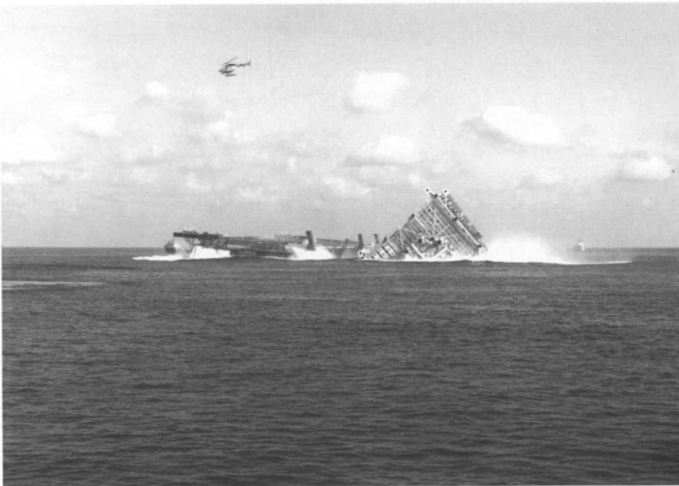
Launching the Lena tower
