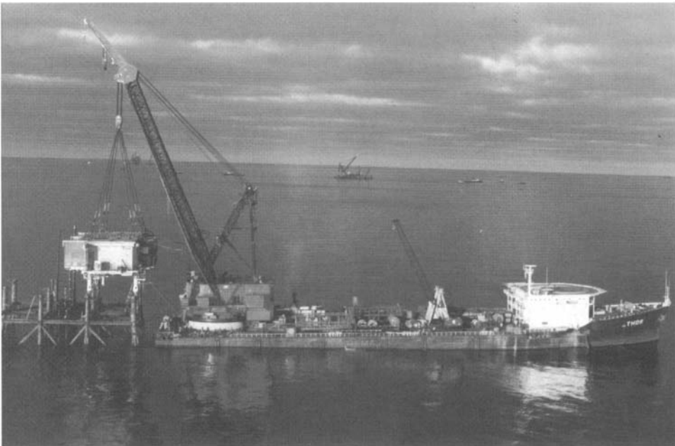
Placing of Forties deck module. Photo courtesy of Dirk Blanken
