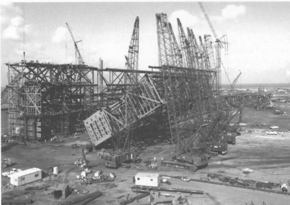
Box roll up of Exxon's Lena tower at Harbor Island
