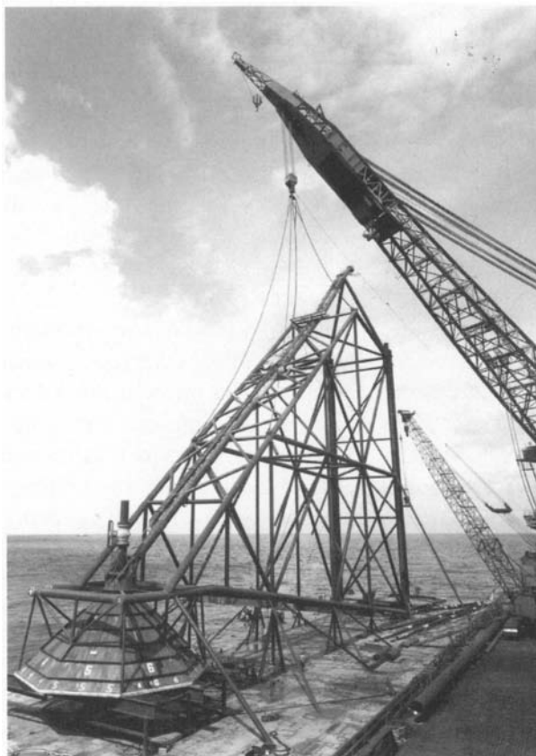
Sombrero and cantilevered boom ready for installation
