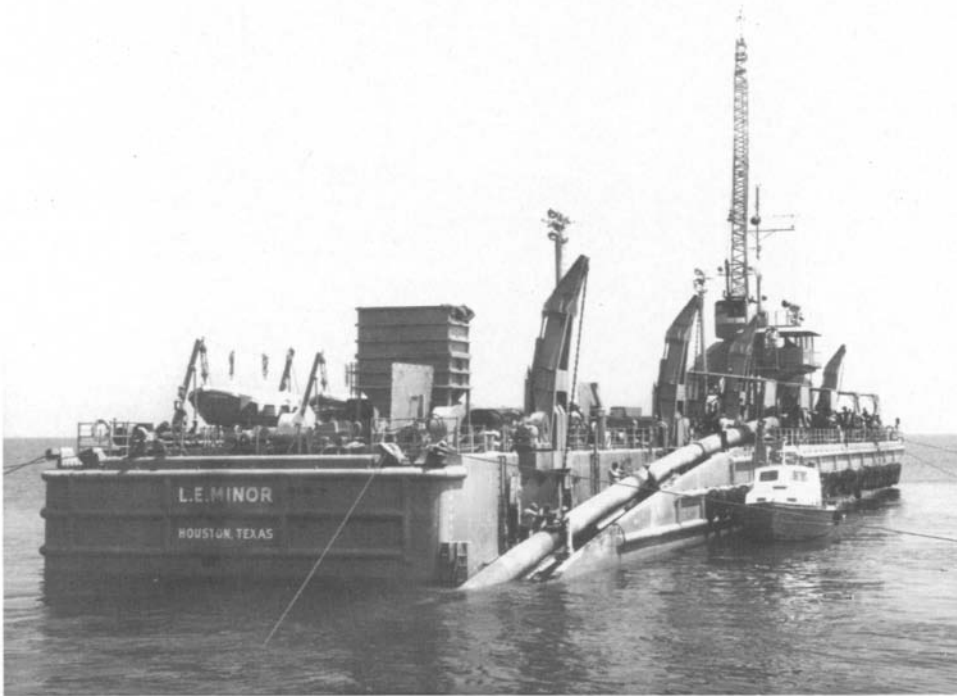
The L.E. Minor pipelaying barge
