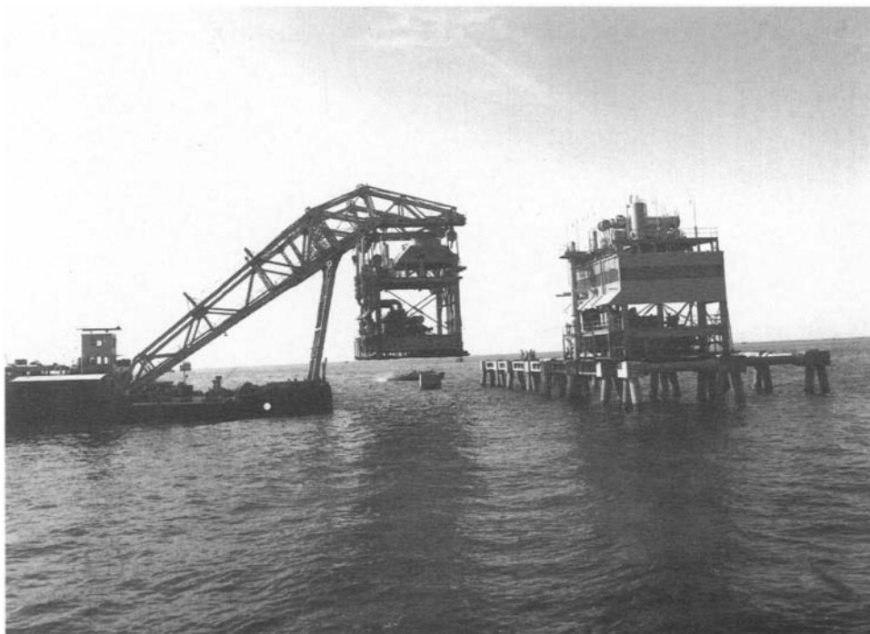
Setting a prefabricated module of the Menegas I
