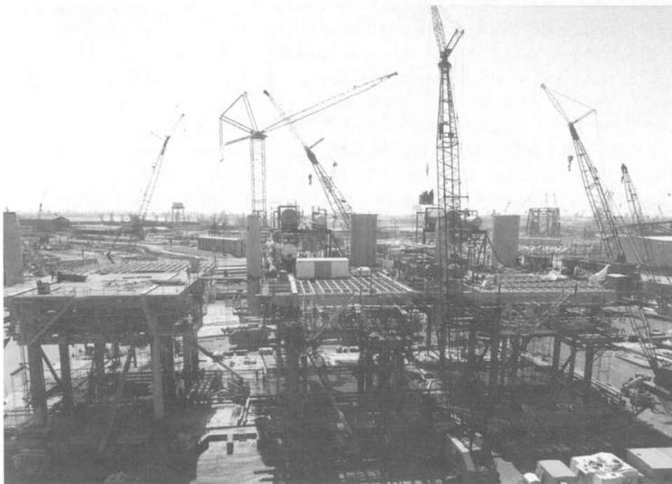
Three PEMEX platforms under fabrication at Greens Bayou
