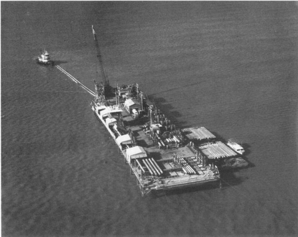
The M-211 pipelaying barge with stinger
