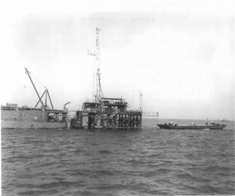
Kermac 16 under construction
