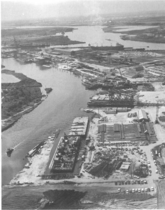
Greens Bayou fabrication yard during the 1960s
