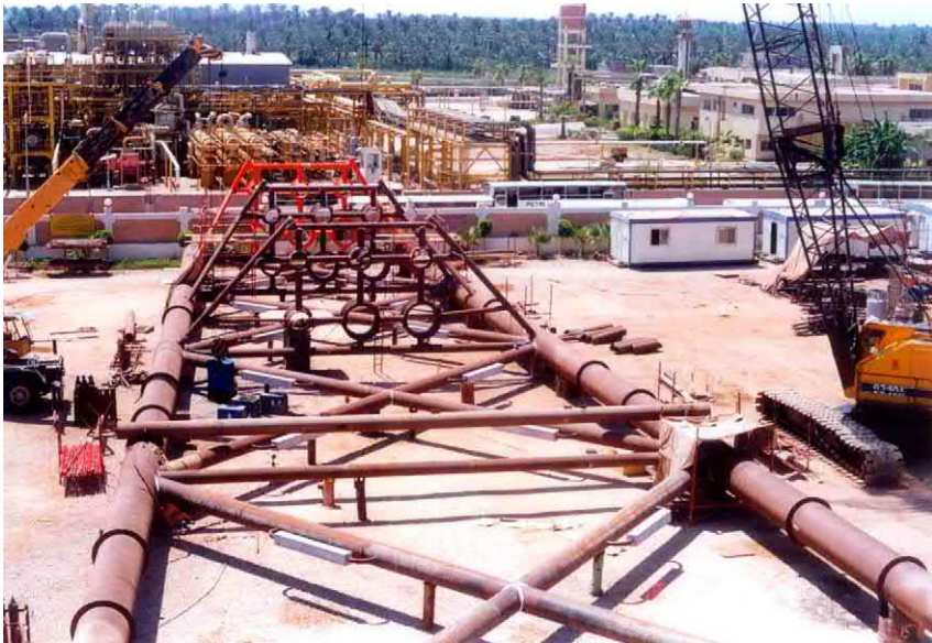
FIGURE 5.24 Fabrication of the last face frame for the jacket.
