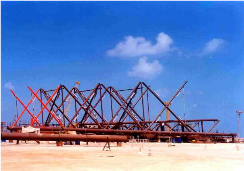
FIGURE 5.21 Erection of X bracing with the horizontal bracing.
