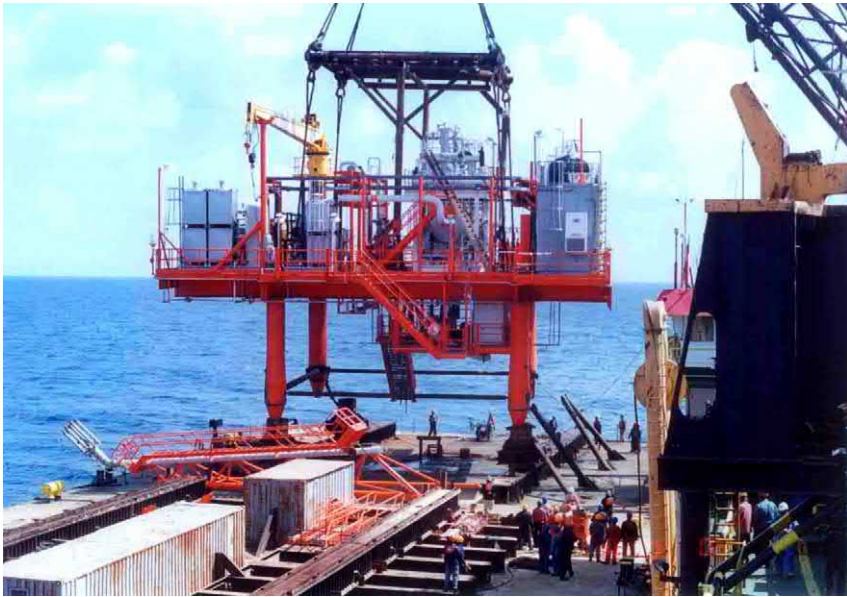
FIGURE 5.27 Transport of the topside to the barge.
