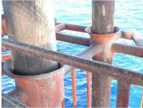
FIGURE 3.21 Conductor guides.
