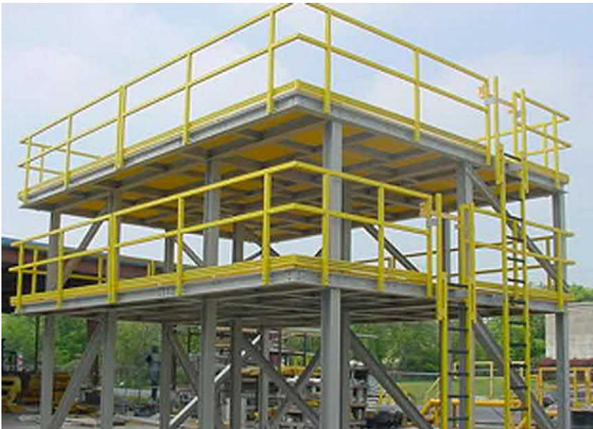
FIGURE 7.43 Deck from FRP.
