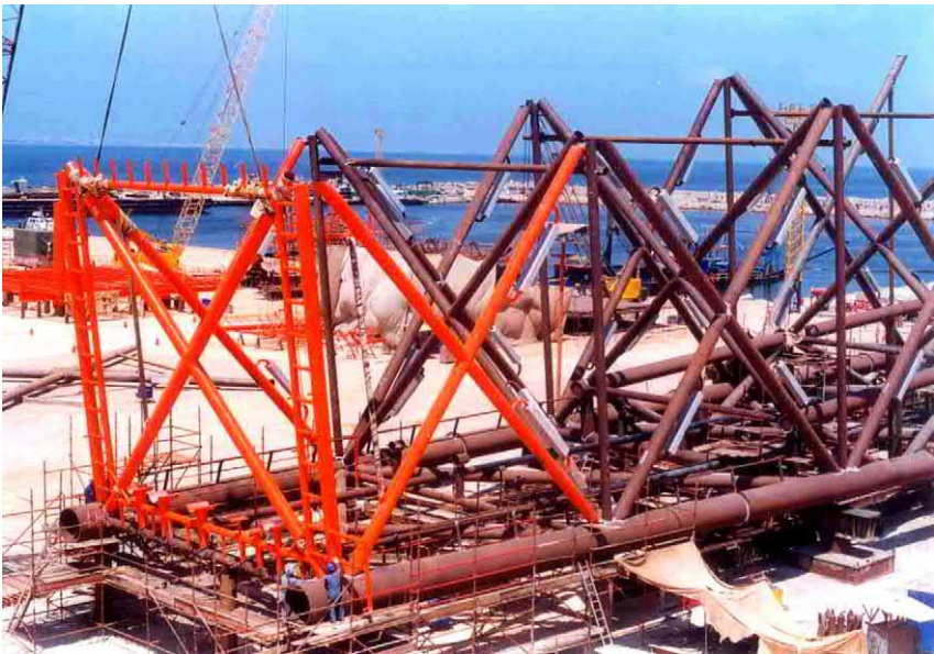
FIGURE 5.22 Erection of the last horizontal level for the jacket.
