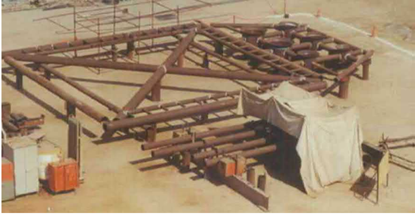
FIGURE 5.23 Fabrication of the conductor guide with the horizontal frame.
