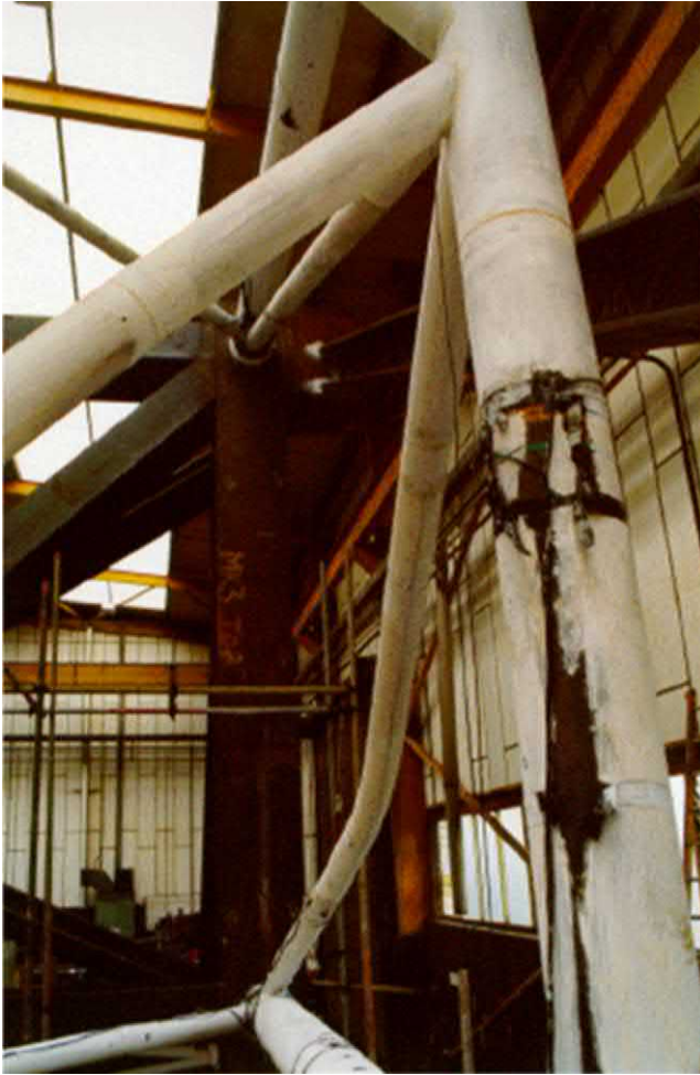
FIGURE 3.10 Buckling in the member for K bracing.
