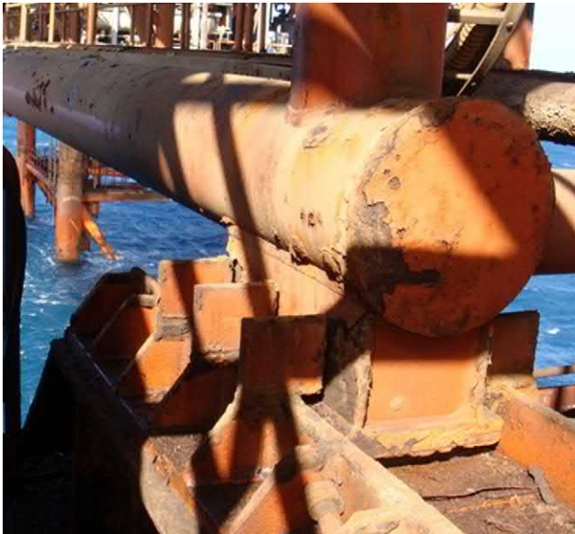
FIGURE 3.59 Roller support for the bridge.
