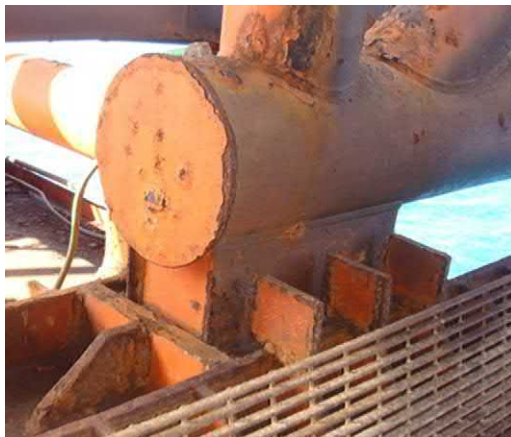
FIGURE 3.58 Hinge support for the bridge.
