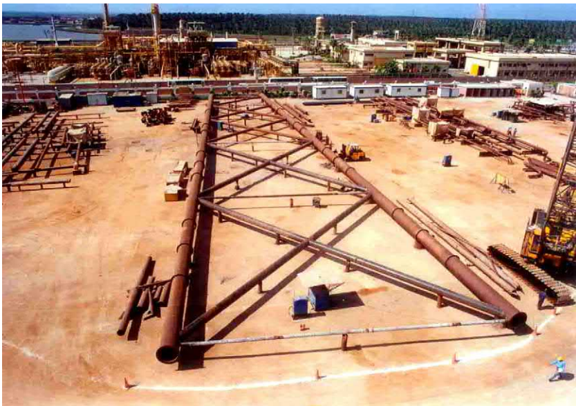
FIGURE 5.17 Frame jacket located horizontally.
