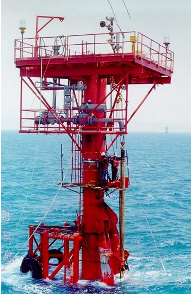
FIGURE 1.9 Photograph of three-legged platform.
