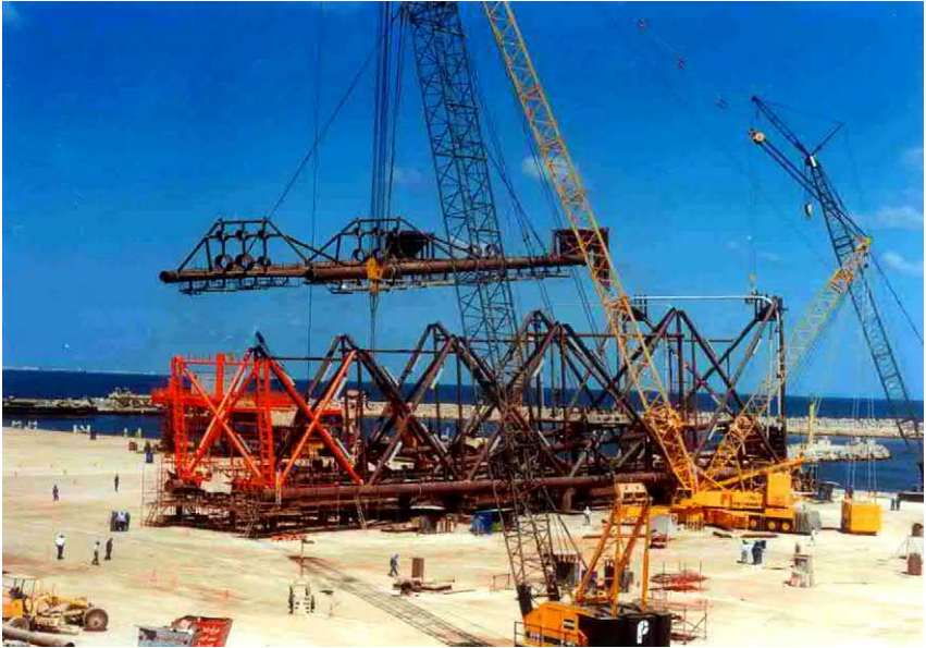
FIGURE 5.25 Erection of the last face of the jacket.
