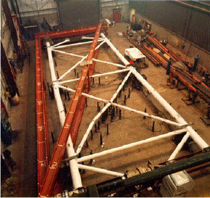
FIGURE 3.8 Buckling of beam in the jacket.
