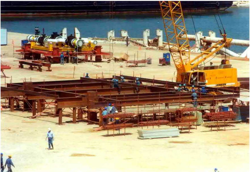
FIGURE 5.26 Fabrication of the topside.
