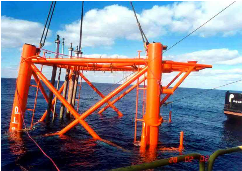
FIGURE 5.48 Lifting the jacket for installation.
