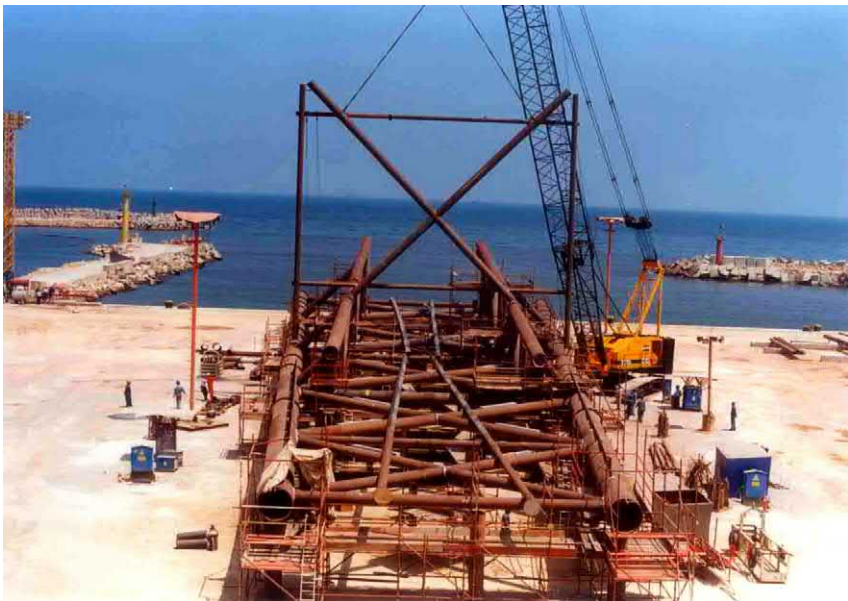
FIGURE 5.20 Start of erection of the horizontal bracing.
