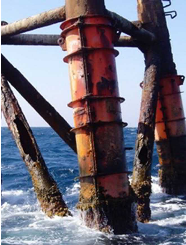
FIGURE 7.47 Corroded bracing.
