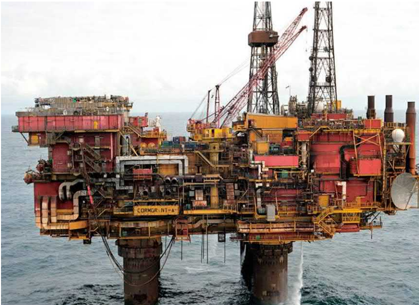
FIGURE 1.6 Concrete gravity platform.
