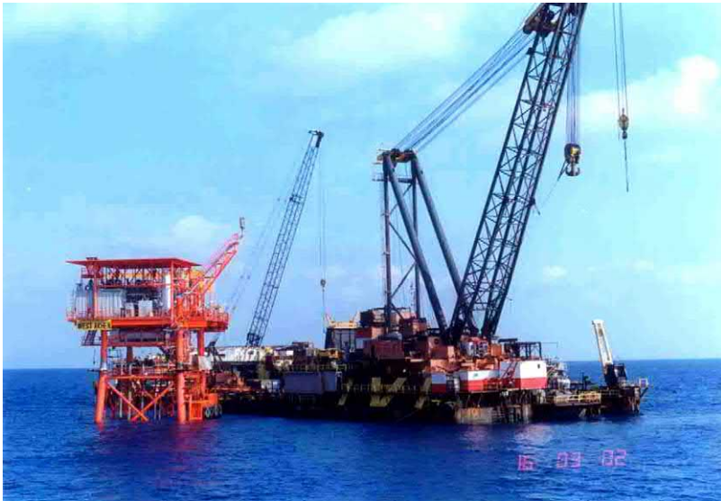
FIGURE 5.47 Crane barge near the platform.
