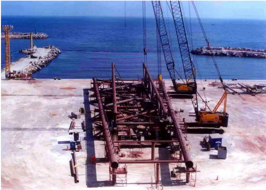
FIGURE 5.19 Erection of strength framing for the launching process.
