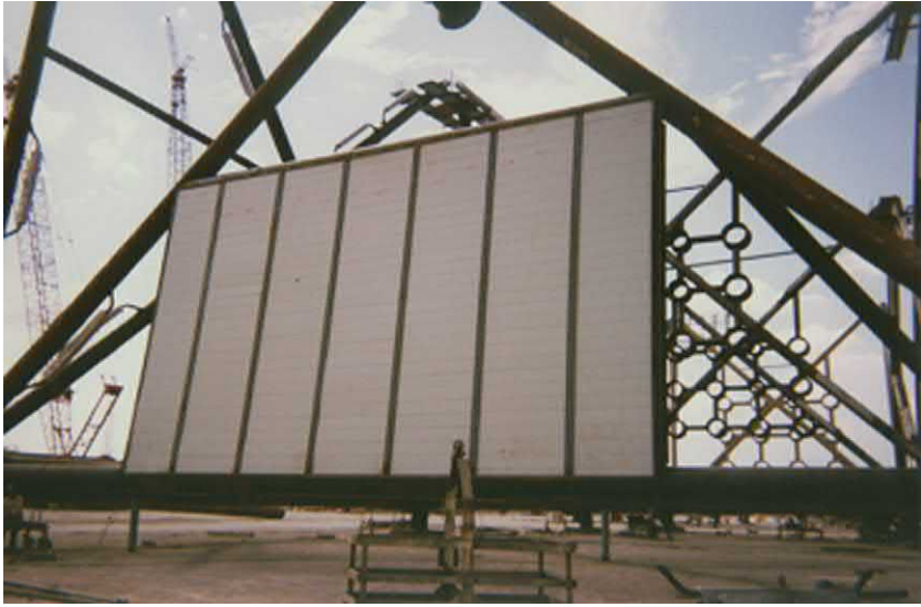
FIGURE 7.46 Fiberglass mud-mat system.
