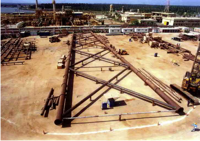
Figure 5.17 Frame jacket located horizontally.
