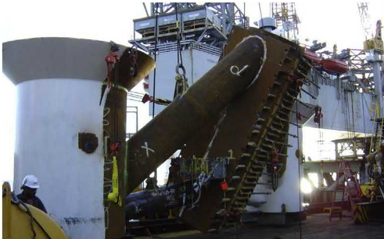
Figure 7.55 A prestressed clamp.
