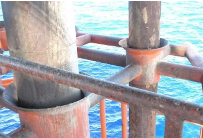
Figure 3.21 Conductor guides.
