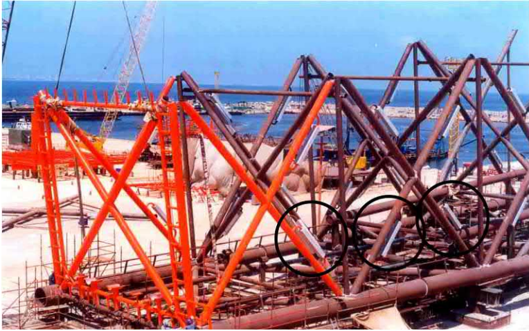
Figure 6.8 Location of the anode in the jacket during construction.
