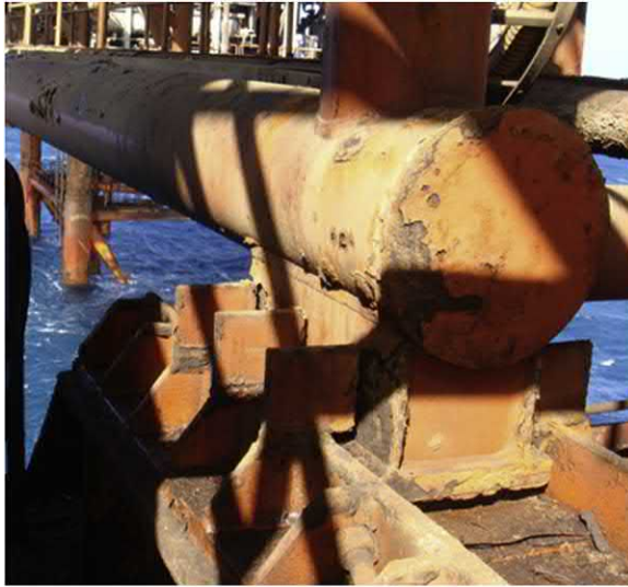
Figure 3.60 Roller support for the bridge.
