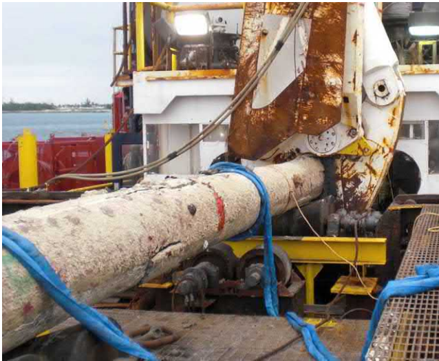
Figure 7.31 Shear cutting on a barge.
