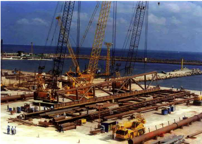
Figure 5.18 (A and B) Erecting the side frame.
