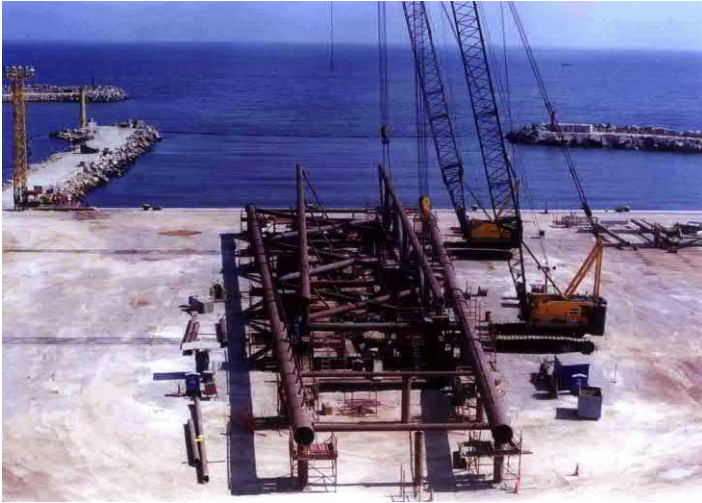
Figure 5.19 Erecting strength framing for the launching process.
