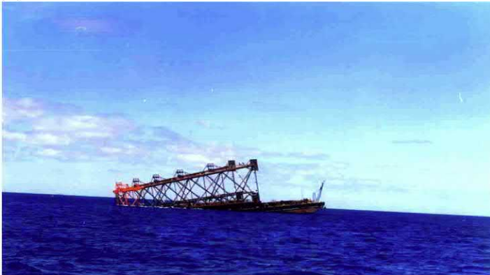
Figure 5.50 (A) Start of launching the jacket; (B) launching the jacket.
