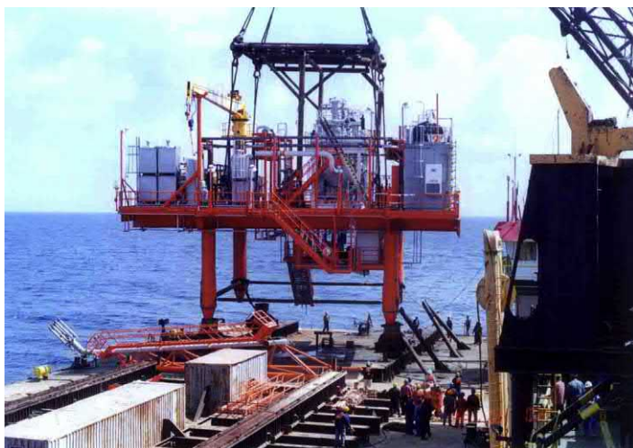
Figure 5.30 Presenting the topside to the barge.
