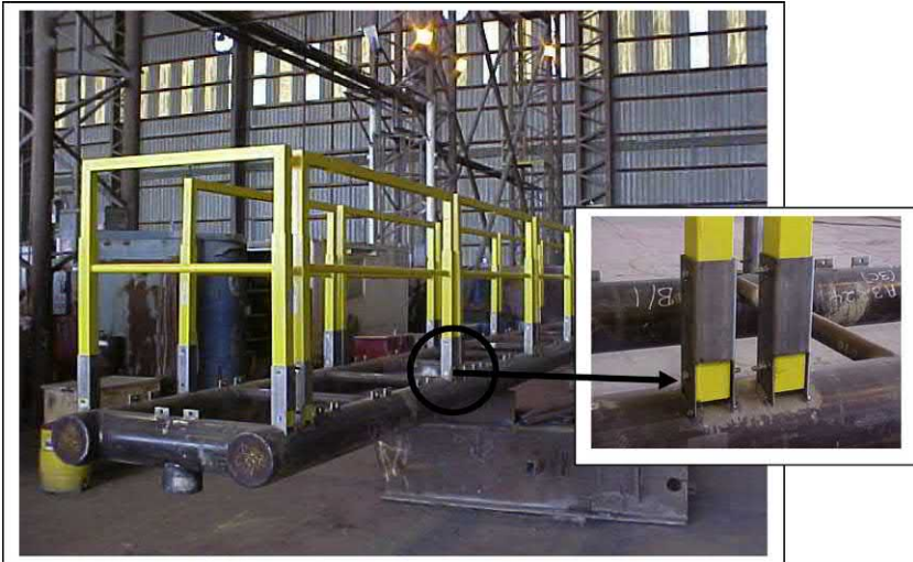
Figure 7.64 Glass fiber reinforced polymer (GFRP) handrails.
