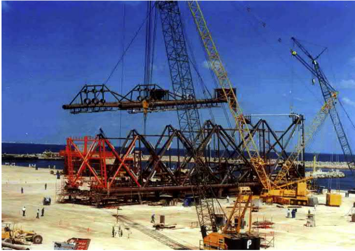
Figure 5.25 Erecting the last face of the jacket.
