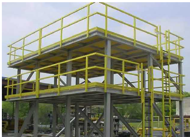
Figure 7.60 An fiber reinforced polymer (FRP) deck.
