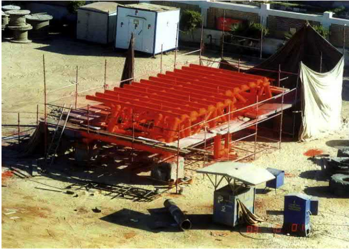
Figure 5.29 Fabricating the boat landing and coating.
