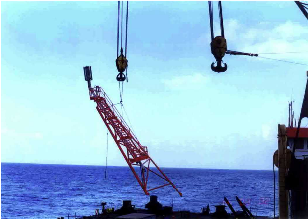
Figure 5.31 Lifting the flare stack to fix to the topside offshore.
