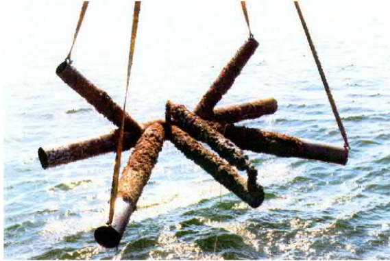
Figure 7.48 Corroded part removal.
