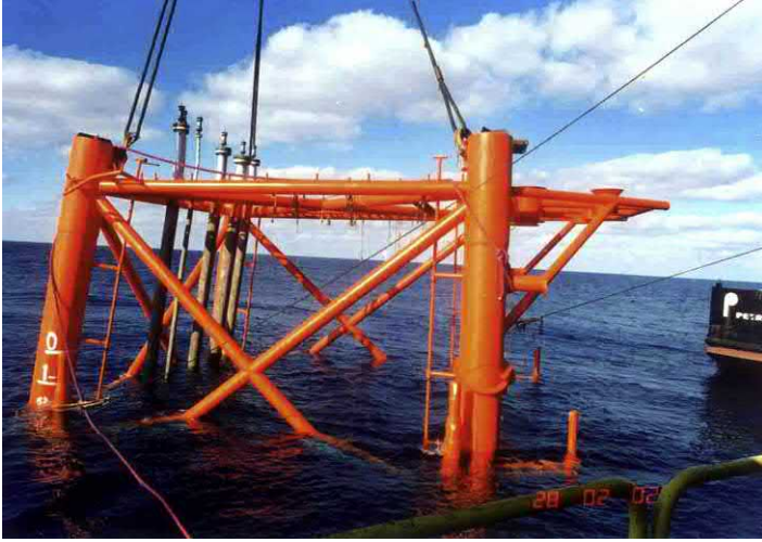
Figure 5.52 Lifting the jacket for installing.
