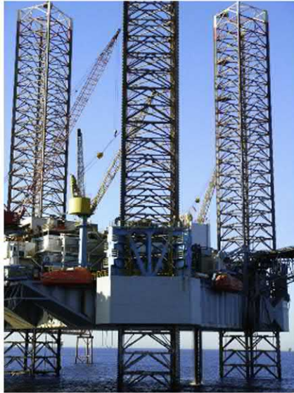
Figure 5.45 (A) Jack-up barge near platform and (B) jack-up barge configuration.
