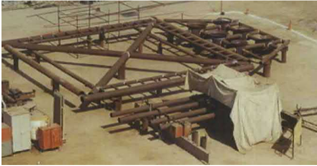
Figure 5.23 Fabricating the conductor guide with the horizontal frame.
