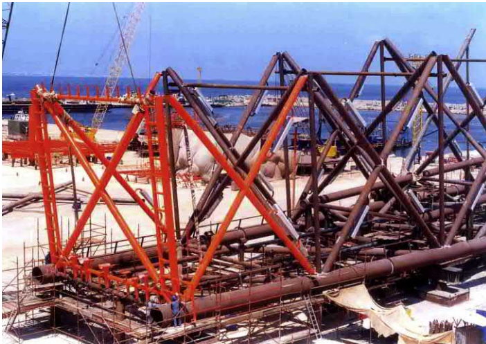
Figure 5.22 Erecting the last horizontal level for the jacket.
