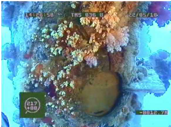
Figure 7.20 Clean detachment of the brace member from the leg.
