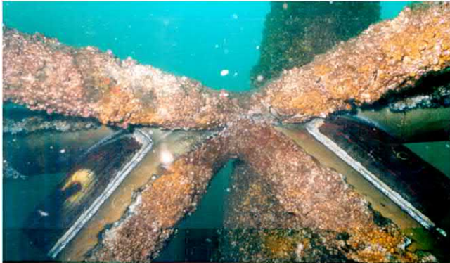
Figure 7.51 Shear pups installed on the platform.
