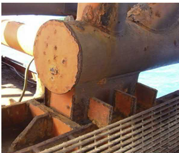
Figure 3.59 Hinge support for the bridge.
