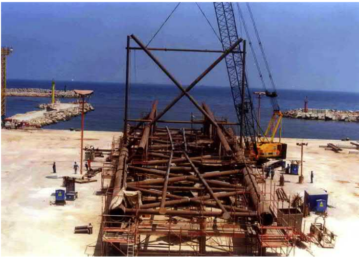
Figure 5.20 Starting erecting the horizontal bracing.
