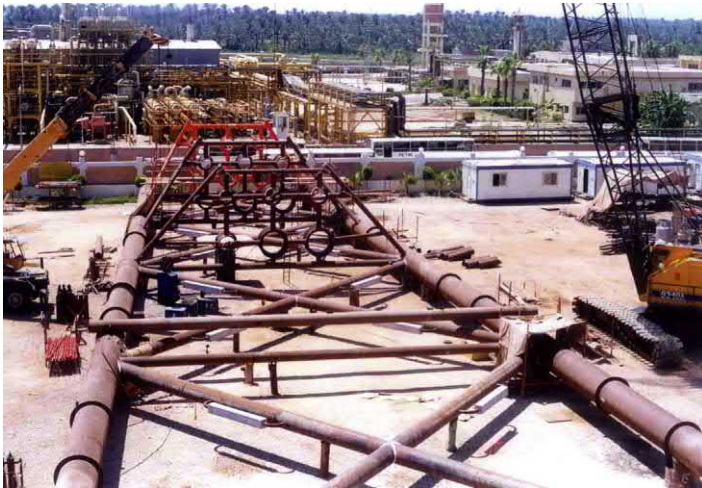
Figure 5.24 Fabricating the last face frame for the jacket.
