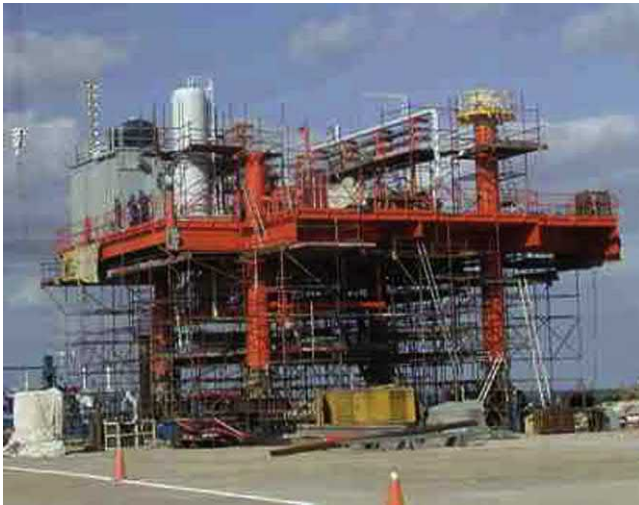
Figure 5.28 Painting the topside after assembly.
