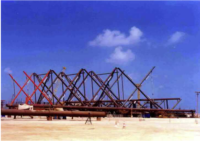
Figure 5.21 Erecting the X bracing with the horizontal bracing.
