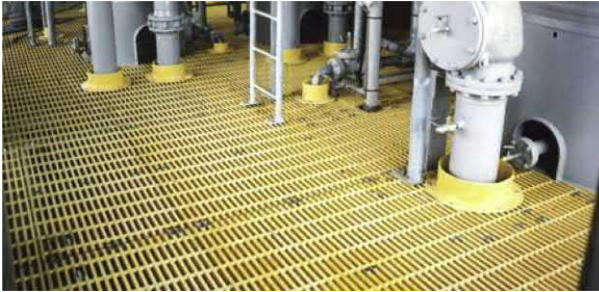
Figure 7.61 Fiber reinforced polymer (FRP) grating.
