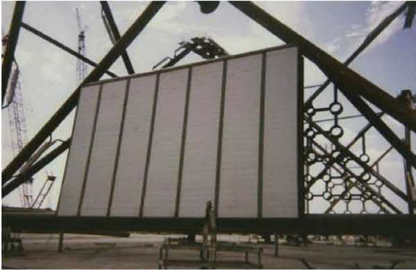
Figure 7.65 Fiber reinforced polymer (FRP) mudmat system.
