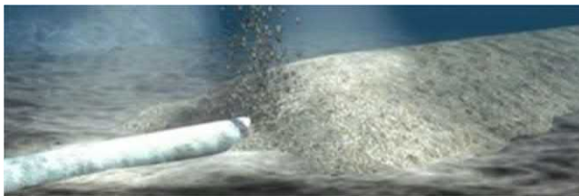
Figure 9.10 Rock dump for stabilization.
