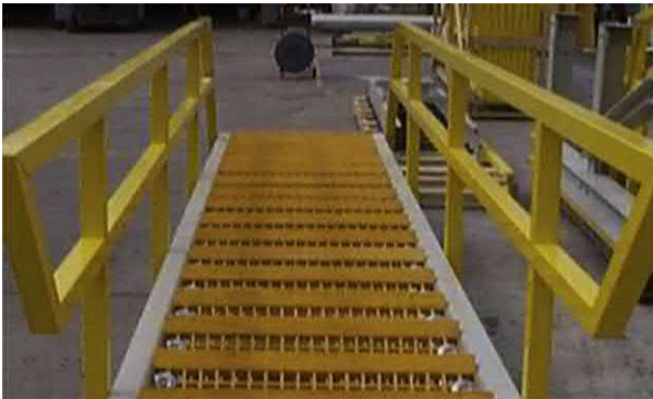
Figure 7.62 Nonwave zone fiberglass stairs.
