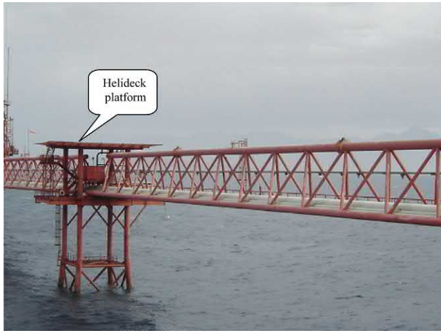
Figure 1.5 Photo of bridges connecting a helideck platform.
