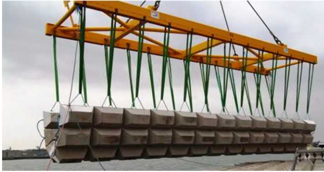
Figure 9.8 Concrete mattress.
