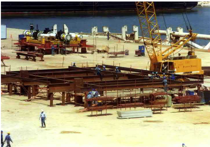
Figure 5.26 Fabrication of the topside.
