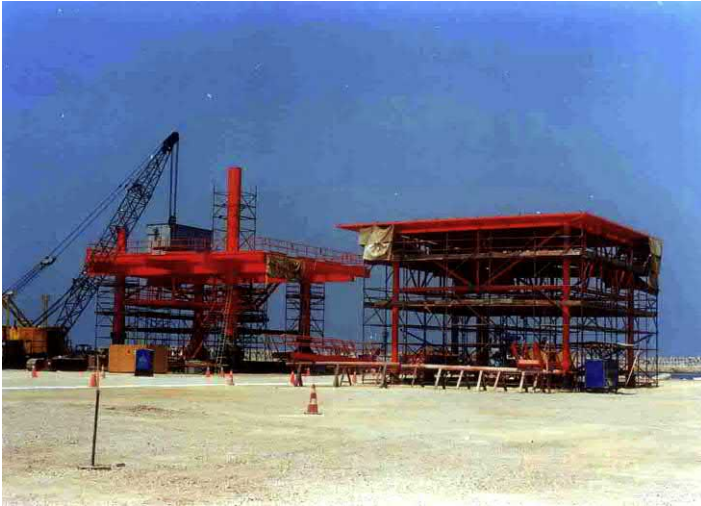
Figure 5.27 Erecting the deck and the helideck.
