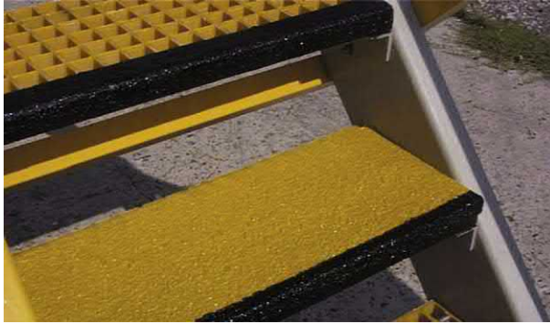
Figure 7.63 Stair tread covers.
