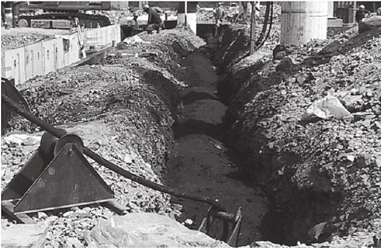
Laying of flexible anode
