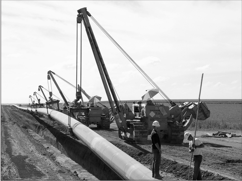
Fig. 8–6. Lowering the pipeline into position ( Source: Miesner and Leffler)
