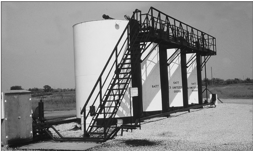
Fig. 8–1. Crude oil stock tanks at a well site ( Source: Hyne, N. J. )
