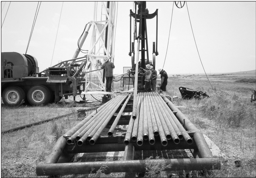
Fig. 5–18. Tubing being run into a well (Source: Hyne, N. J.)
