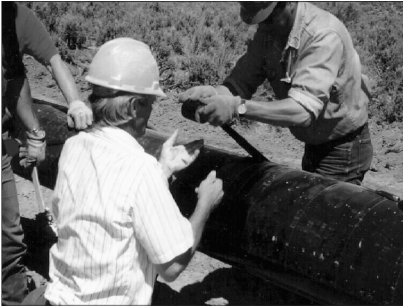
Fig. 8–5. Applying spiral-wrap tape to a pipe (Source: Miesner and Leffler)
