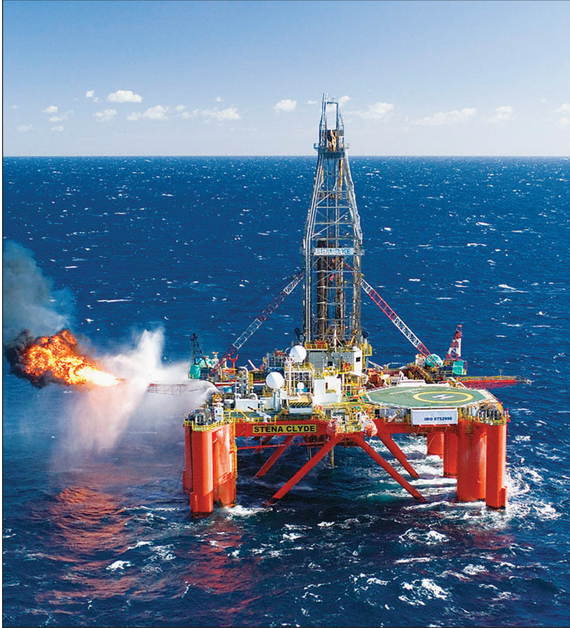
Fig. 6–2. Semisubmersible rig (Source: Oil & Gas Journal )
