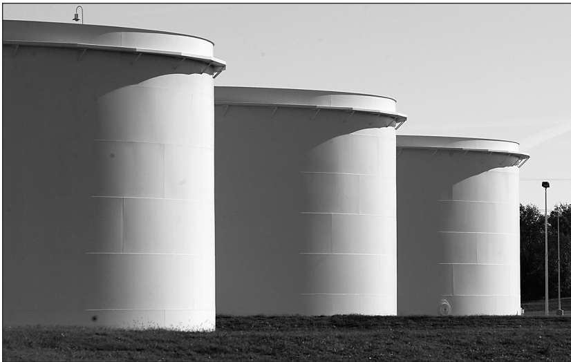
Fig. 8–16. Oil storage tanks (Source: Miesner and Leffler)
