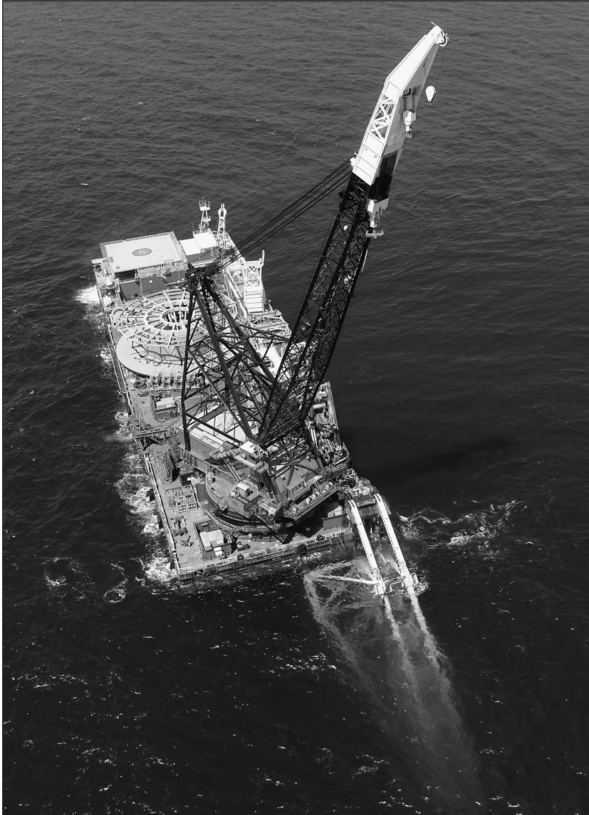
Fig. 8–14. Reel barge laying pipeline offshore (Source: Miesner and Leffler)
