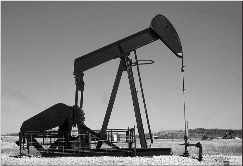
Fig. 7-1. Sucker-rod pumping unit (Source: Hyne, N. J.)
