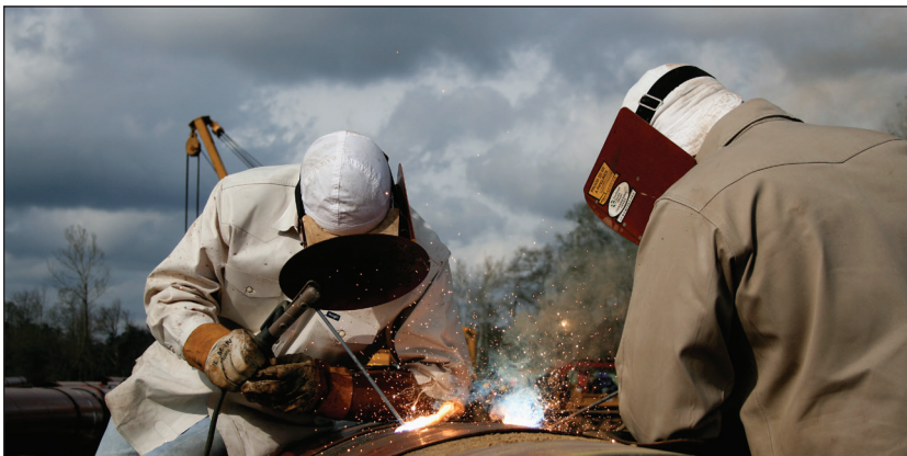
Fig. 8–4. Manual pipeline welding ( Source: Oil & Gas Journal )
