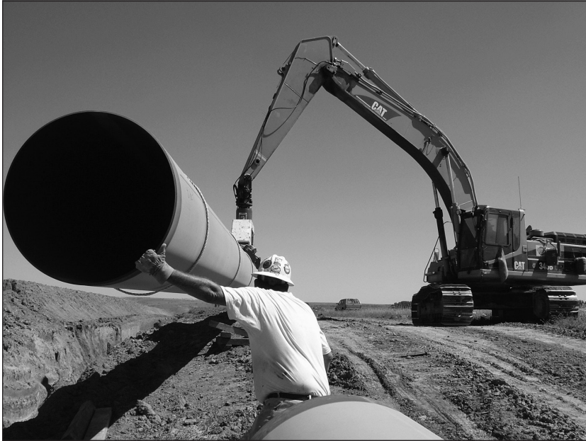
Fig. 8–3. Pipeline sections positioned along the route ( Source: Miesner and Leffler )
