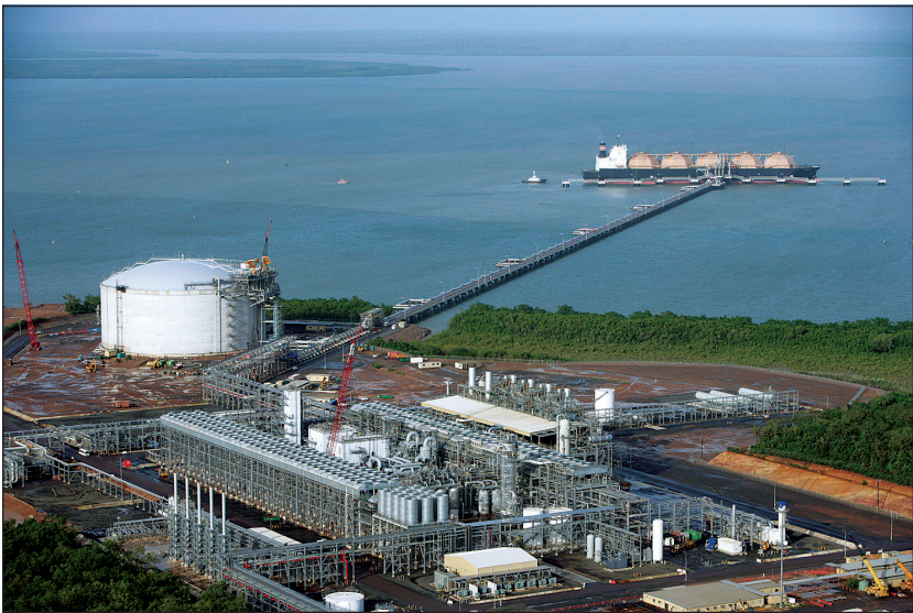
Fig. 10–4. Darwin LNG plant, at Wickham Point, Australia (Source: Oil & Gas Journal )
