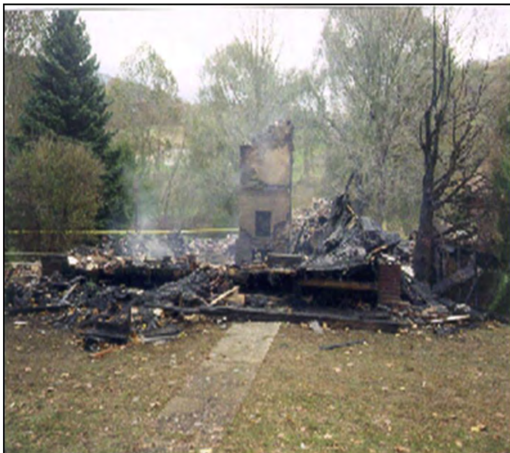
FIGURE 4.2 1999: Photograph showing the remains of a residence after an explosion caused by the migration of stray combustible gas. The investigation revealed the migration of stray gas was due to underground coal mining.
