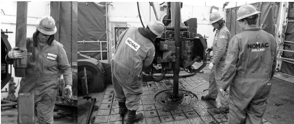
Fig. 1-7 Drill pipe connection
