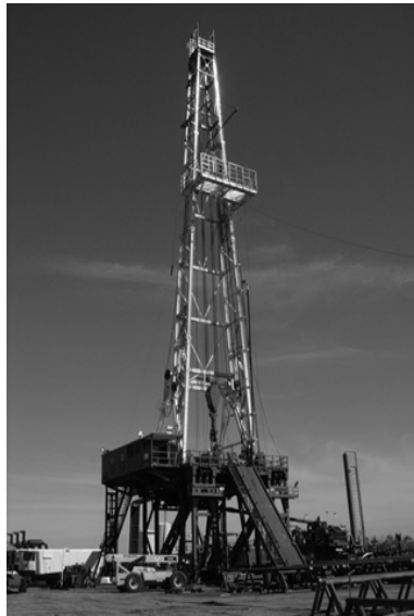
Fig. 1-1 Rotary drilling rig
