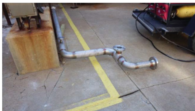
Figure 10.15 20-foot replacement piping (Source: csb.gov).
