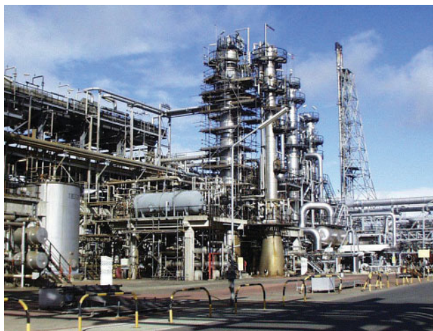
Figure 12.30 Adip Regenerators and Sour Water Strippers. (Courtesy of Honeywell UniSim Design R443, all rights reserved), Honeywell (R) and UniSim (R) are registered trademarks of Honeywell International Inc.
