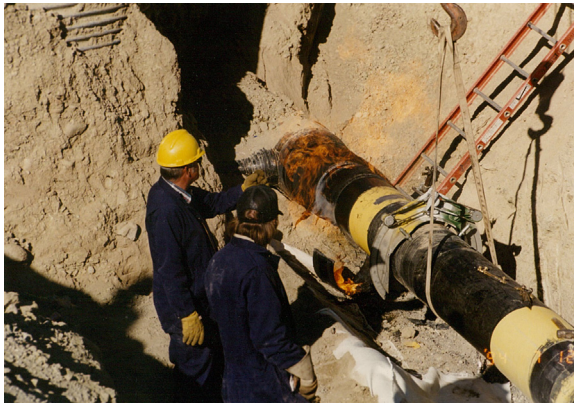
Figure 6.38 Bell hole in a hot ditch.
