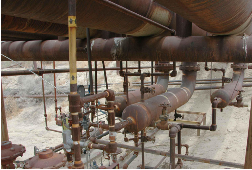
Figure 4.12 Oxygen corrosion.
