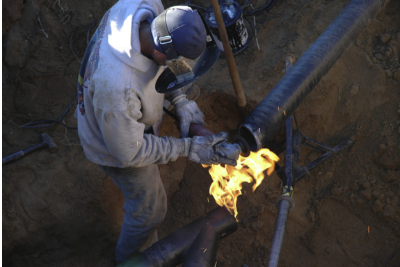
Figure 6.28 Preparing a pipe for welding.
