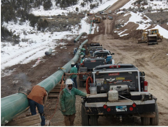
Figure 6.36 Firing-line welding.
