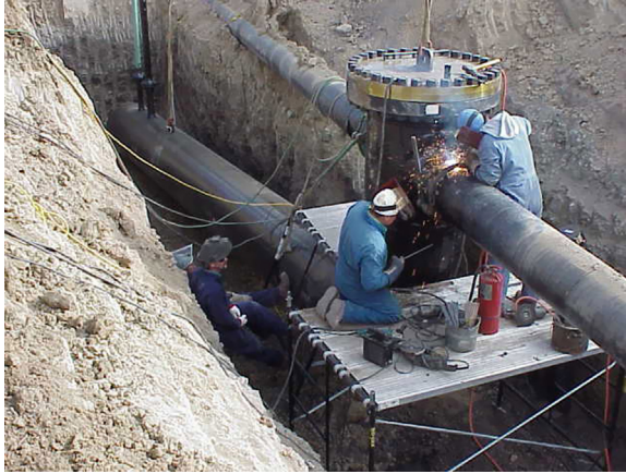
Figure 6.37 Tie-in welds.
