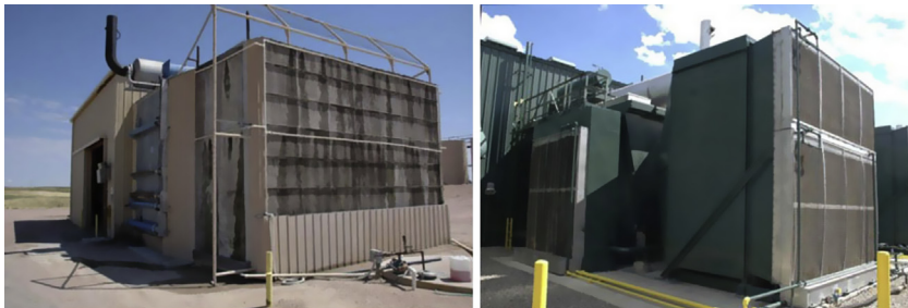
Figure 7.20 Evaporative coolers.
