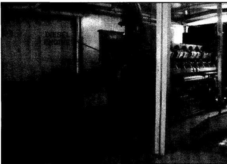
Figure 81. The diesel engine at right drives the electric generator attached directly to the engine. This engine-generator set is one of three on this rig.
