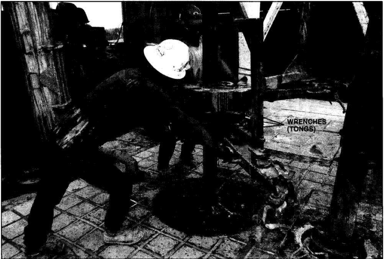
Figure 46. Two rotary helpers latch big wrenches (tongs) onto the drill pipe.
