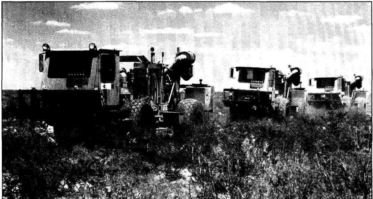
Figure 58. Several special trucks vibrate plates against the ground.
