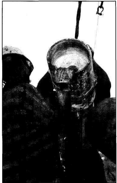
Figure 168. Crew members install a float collar into the casing string.
