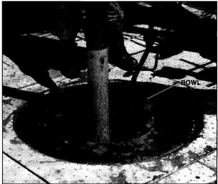
Figure 102. Crew members are installing one of two halves that make up the tapered bowl.
