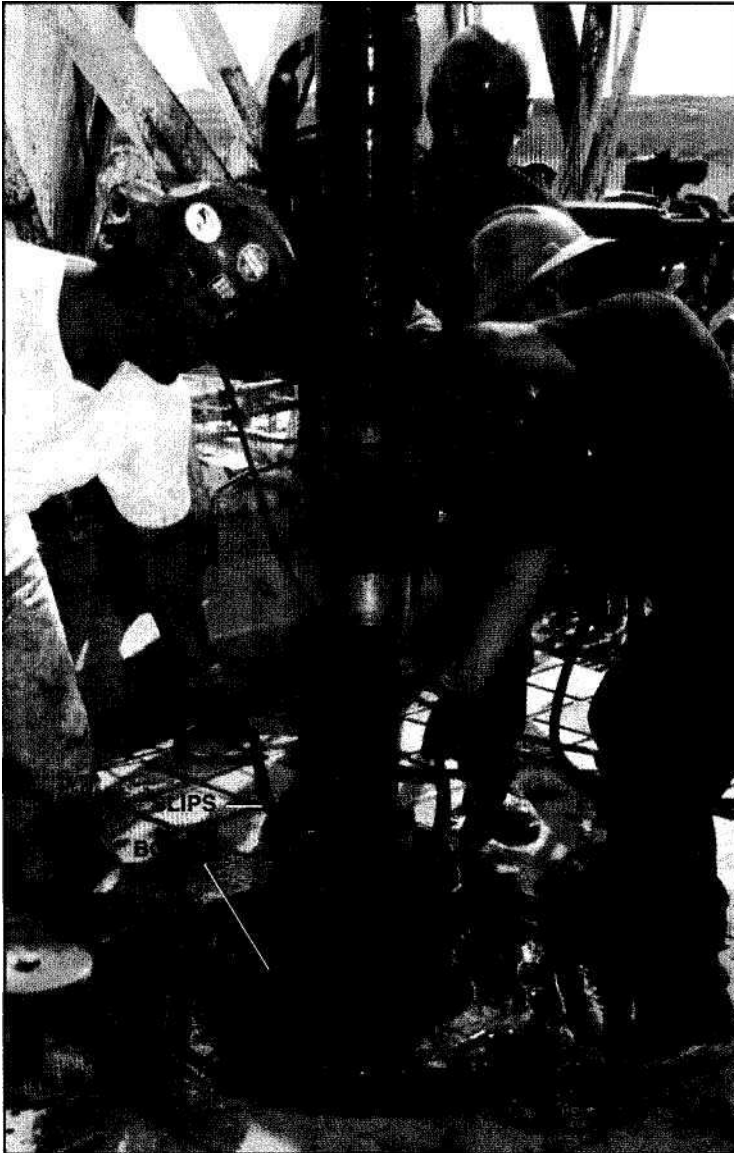
Figure 103. Crew members set slips around the drill pipe and inside the master bushing's tapered bowl to suspend the pipe.
