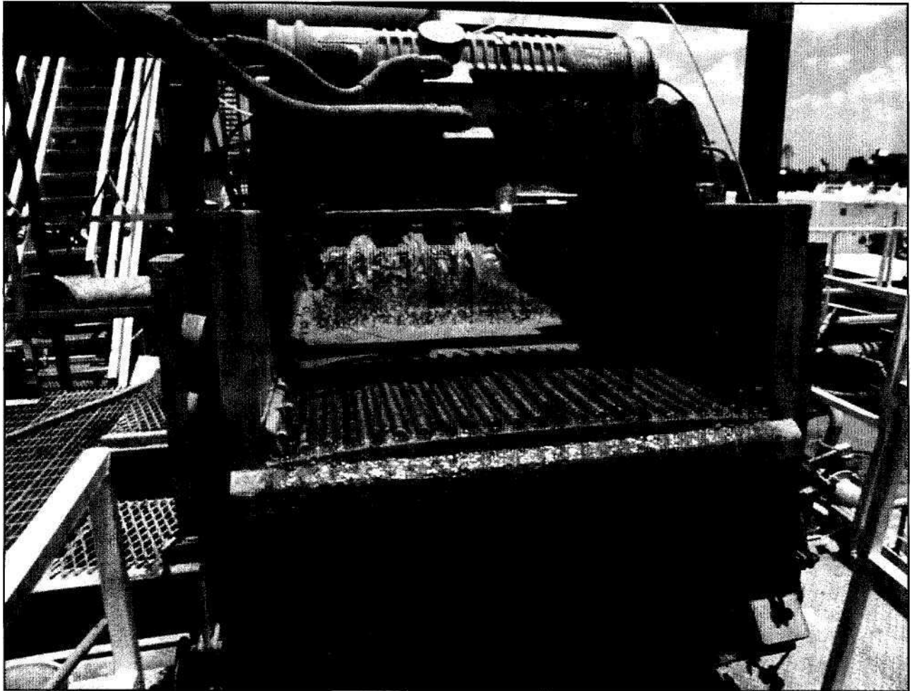
Figure 12p. Mud and cuttings fall onto the shale shaker, which removes the cuttings. The mud falls into a tank below the shaker.
