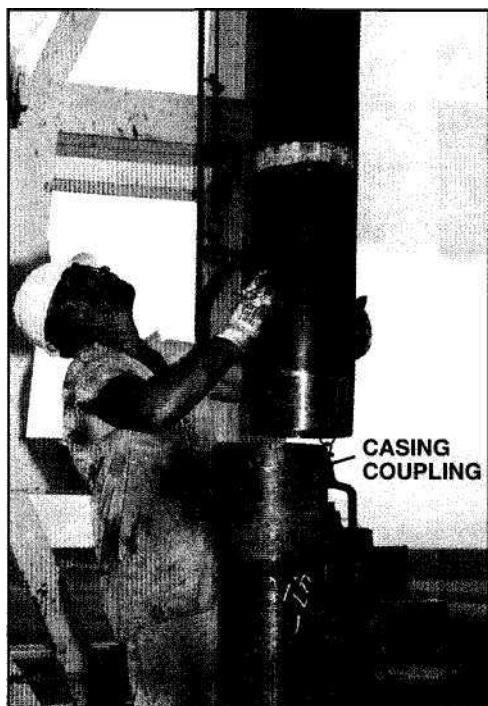
Figure 4.1. This member of a casing crew is stabbing one joint of casing into another. The red fitting is a casing coupling used to connect the joints.
