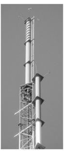
FIGURE 2.4.8 Antenna installation using top-mounted and side-mounted antennas. (Photo courtesy of Electronics Research, Inc. (ERI).)
