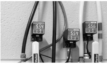
$FIGURE \ 6.7.16 \ \ Electronic \ pressure \ gauges \ can \ allow \ direct \ psi \ readings \ on \ the \ remote \ control.$
