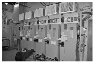
FIGURE 6.7.44 Transmitter room with five HVAC units for redundancy.
