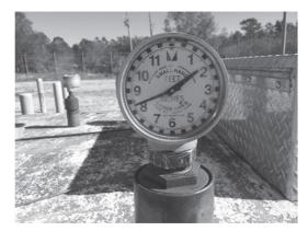
FIGURE 6.7.24 Generator fuel tank gauge.
