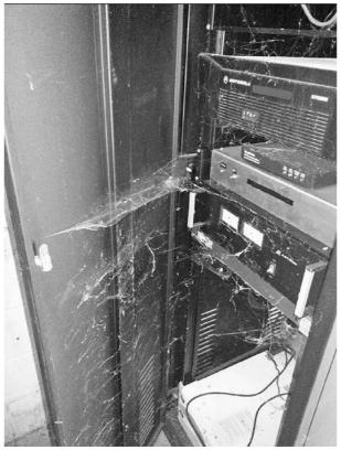
FIGURE 6.7.2 Neglected transmitter site equipment.
