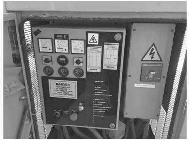
FIGURE 6.7.22 Main circuit breaker on a generator.
