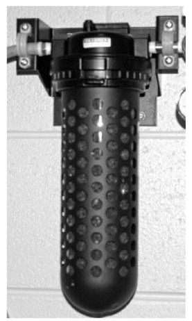
FIGURE 6.7.18 Dryer module on a nitrogen generator.
