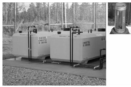
FIGURE 6.7.25 Double-walled fuel tank (left) and leak detect gauge (right).
