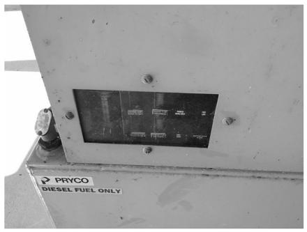
FIGURE 6.7.27 Generator day tank and fuel gauge
