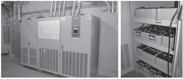
FIGURE 6.7.48 Large UPS to power a transmitter and supporting equipment.
