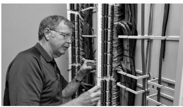
FIGURE 6.3.13 Rack wire management and cable termination. (Courtesy: WISH-TV.)
