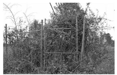
FIGURE 6.7.53 Overgrown guy wire anchor should be cleared out immediately.
