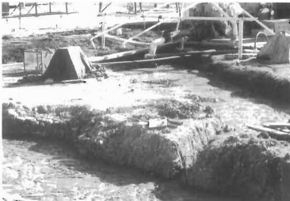
Earthen Pit Design. The earthen pit system was designed as a settling pit that overflowed through a ditch into the suction pit. A duplex mud pump suction is shown at the far end of the suction pit. Drilled solids levels were poorly controlled. Mud treatment consisted of dilution to decrease the drilled solids concentration and viscosity. Fortunately, the well was normally pressured and was easy to drill.
