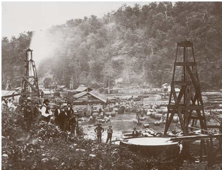
Fig. 1.3 A Pennsylvania oil field in 1862. The two wells shown are the Phillips well and the Woodford well, among the most productive of the time. Note the small distance between them. In the middle of the photo are wooden barrels in which the crude was stored. The size of a barrel was not standardized yet, so the barrels shown are of different sizes
