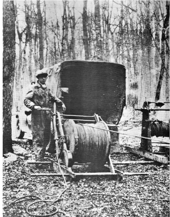
Fig. 13.9 First well logging operations: Pechelbronn Field, Alsace-Lorraine, France. Note multiple winches (from [13.10], courtesy of SPWLA)
