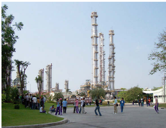
Fig. 20.8 PTT natural gas processing plant in Map Ta Phut, Rayong, Thailand
