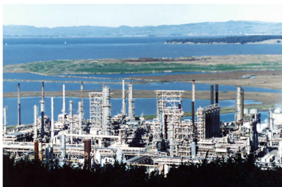
Fig. 34.7 Chevron's Richmond Refinery Lube Oil Plant
