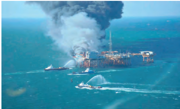
FIGURE 6.10.20 Black Elk Energy's West Delta 32 field exploded and burned following a welding accident in 2012.
