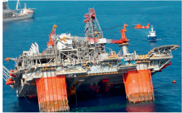
FIGURE 6.10.19 Thunder Horse Platform, found listing after the passage of hurricane Dennis (2005). Source: Wikipedia / US Coast Guard, approved for re-use.
