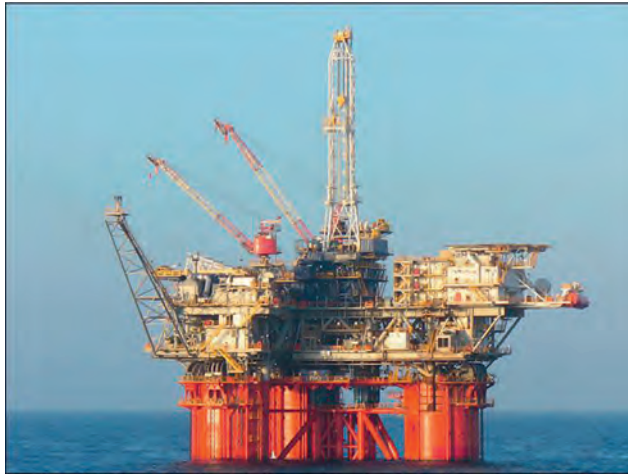
FIGURE 6.10.10 Bennett’s “Mindoc” spar design was utilized for the Telemark hub, installed by ATP [2].
